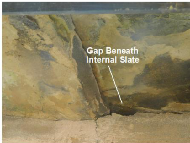
PHOTO 11 Internal View of Western Wall
