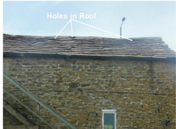
PHOTO 6 View of Northern Roof
