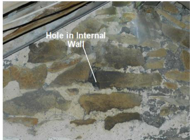
PHOTO 12 Internal View of Southern Wall
