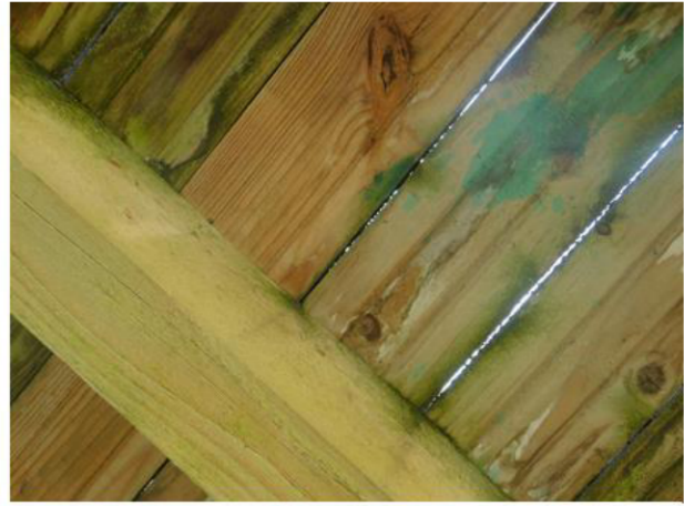
PHOTO 8 Underside of Stairs
