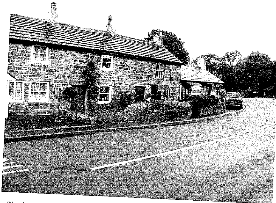
Photo 2 – Cottage row and view of buildings attached to the property
