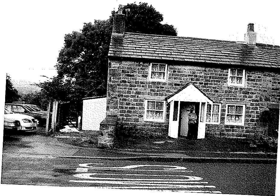
Photo 1 – Front elevation of 6 Whalley Road
