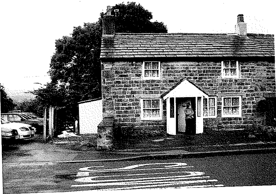
Photo 1 – Front elevation of 6 Whalley Road
