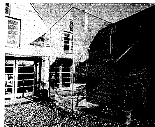
Extension to 16th century Grade 11* listed farmhouse
