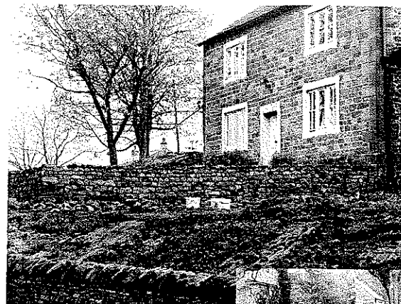
Existing stone walls, in the process of being rebuilt
