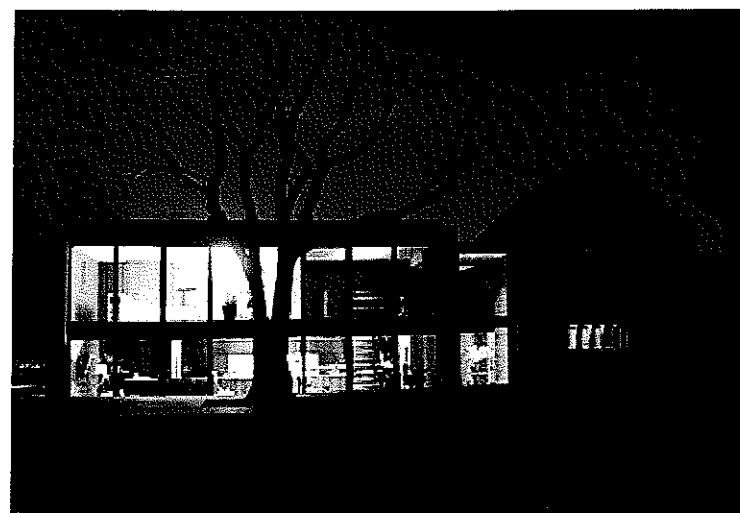
Extension to Oak Farm 17th century farmhouse
