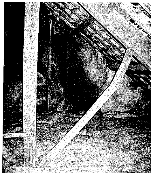
Damp penetration to west wall and broken roof strut
