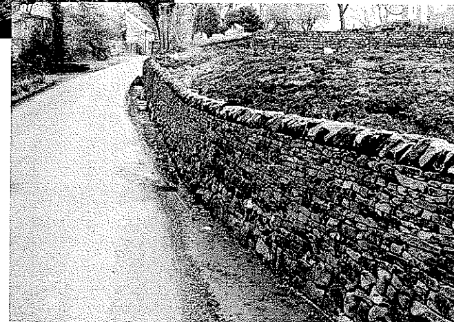
The start of the repair of the boundary stone walls.
