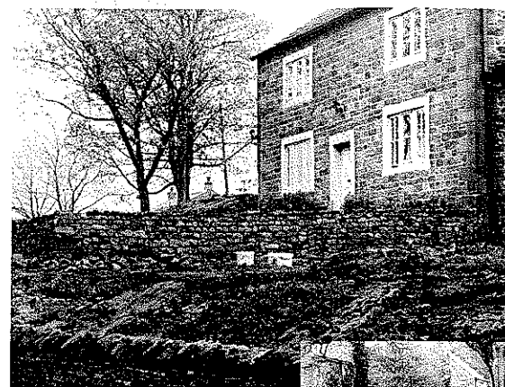
Existing stone walls, in the process of being rebuilt.
