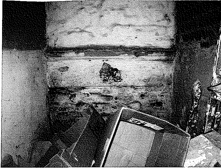
PI. 2 Photograph showing the front of the original range opening.
