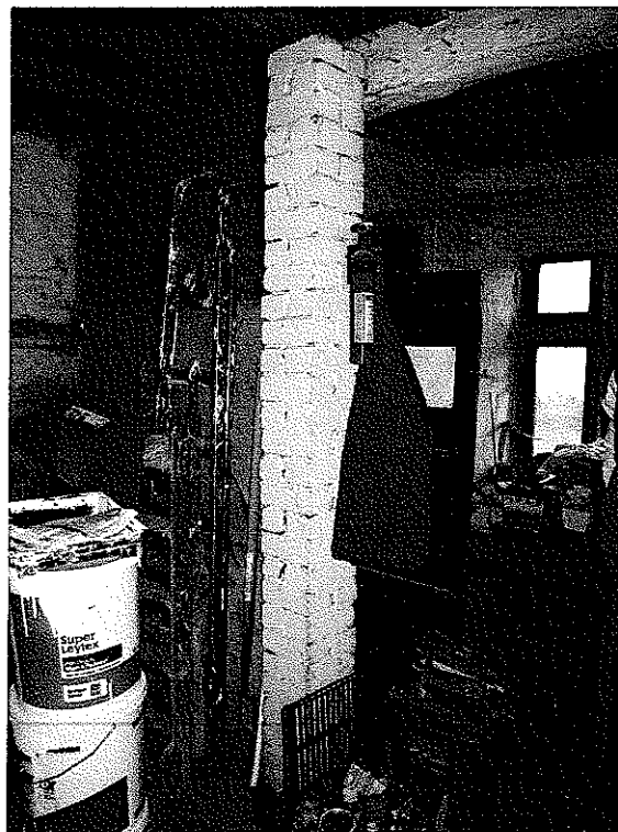
PI. 3 Photograph showing a view of the former kitchen and front windows.
