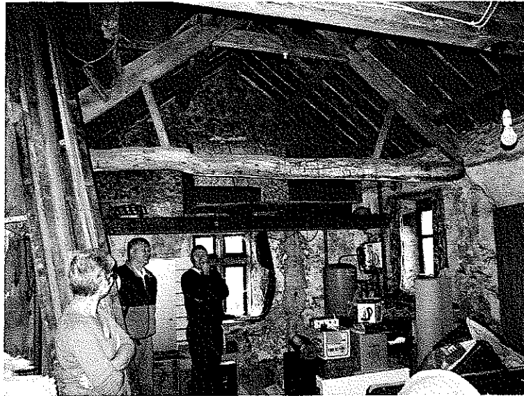
Pl. 6 Photograph showing the bedroom over the kitchen and utility room with part of the plumbing system in the far right hand corner.
