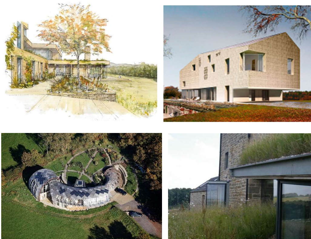
Fig 8. above (clockwise from top left): Examples of approved country houses at Icomb, Cotswold AONB; Mines Park, Cambridgeshire; The Paise, North Pennines AONB; and, The Fossil House, Blackdown Hills AONB
