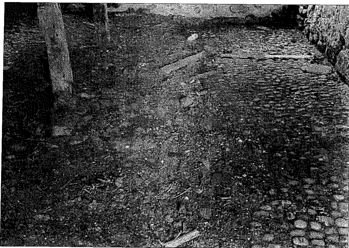
Photo 38: Cobbled floor in added four-stall stable, from the north-east
