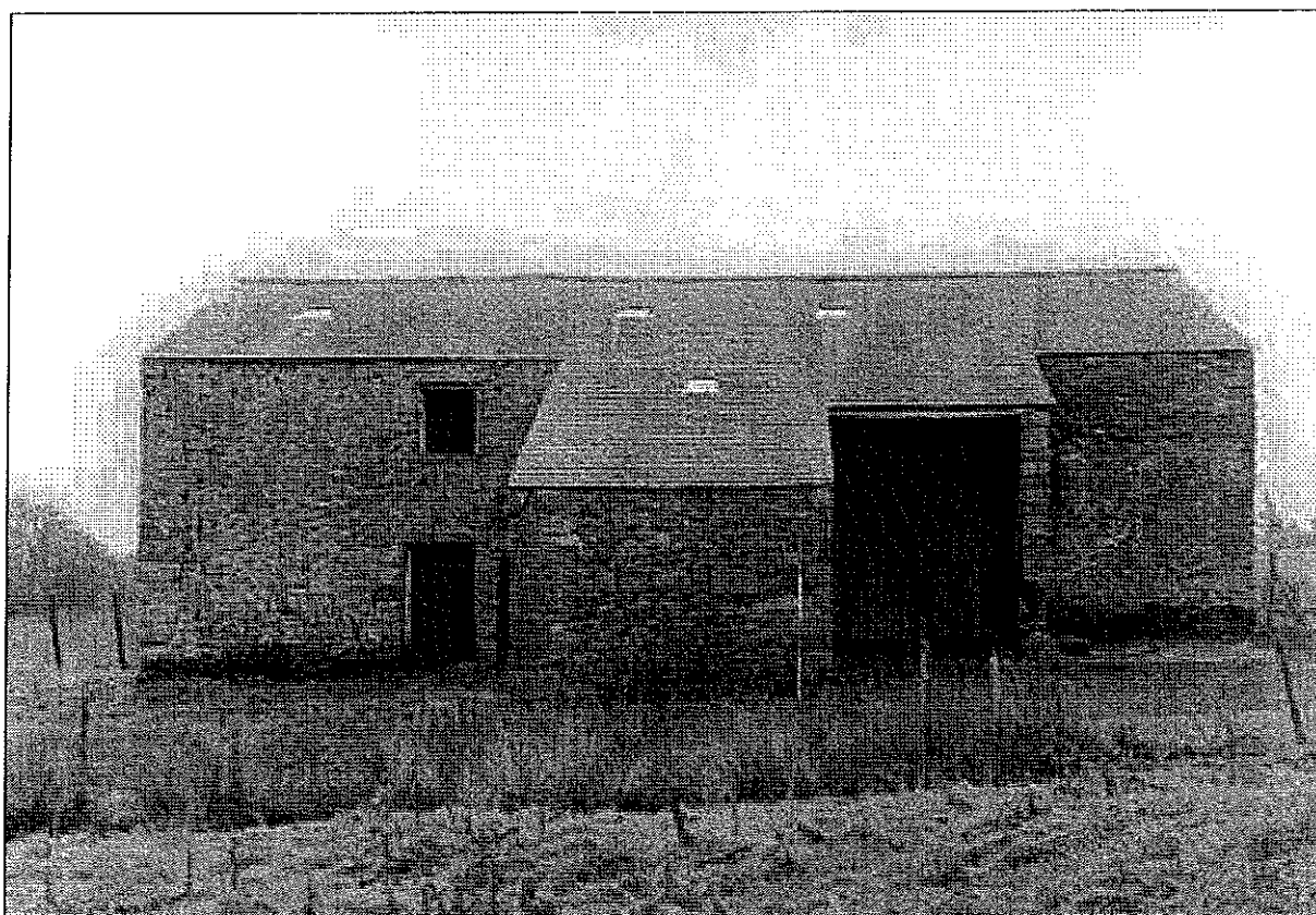
Photo 2: The barn, from the north-east
