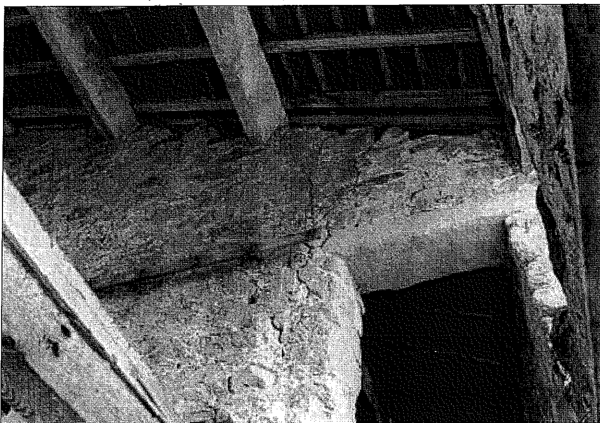
Photo 16: First floor of added stable: coat hooks and doorway to barn
