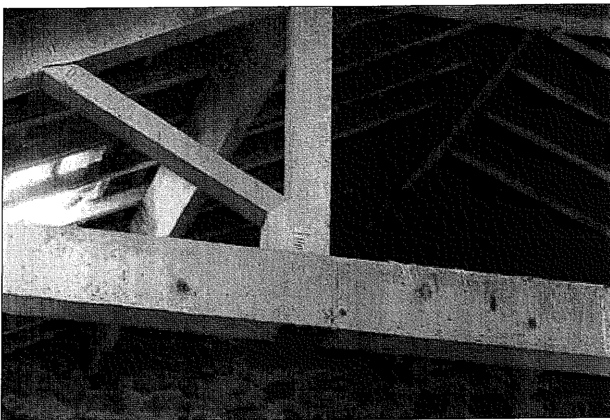
Photo 30: Detail of queen strut, showing numbering on timbers
