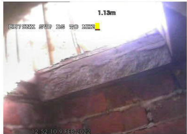
4-1-2A, 00:00:09, 1.13 m Finish manhole, MH2, the pipe is flowing fine
