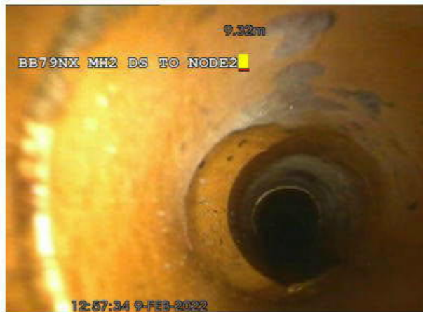
6-1-6A, 00:00:43, 9.39 m Junction at 9 o'clock, diameter: 100mm, PIPELINE FROM MH1
