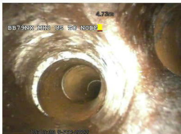
8-1-2A, 00:00:21, 4.73 m Junction at 2 o'clock, diameter: 100mm
