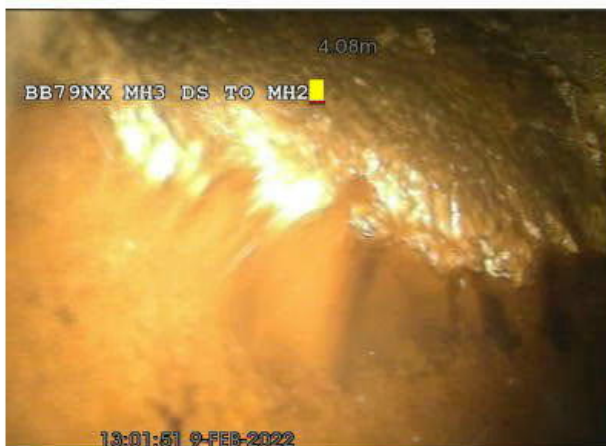
7-1-3A, 00:00:40, 4.08 m Finish manhole, MH2, the pipe is flowing fine
