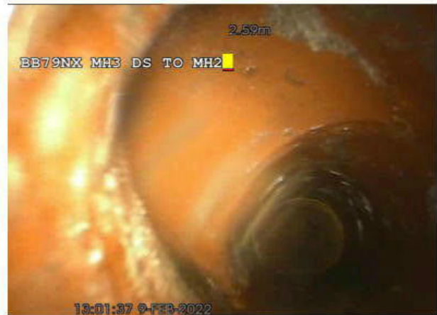
7-1-2A, 00:00:26, 2.59 m Junction at 10 o'clock, diameter: 100mm
