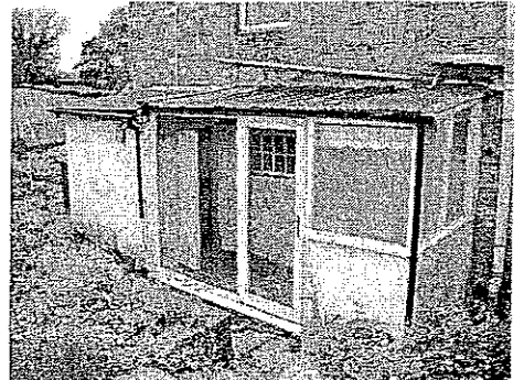
Figure 9: Lean-to at rear of property
