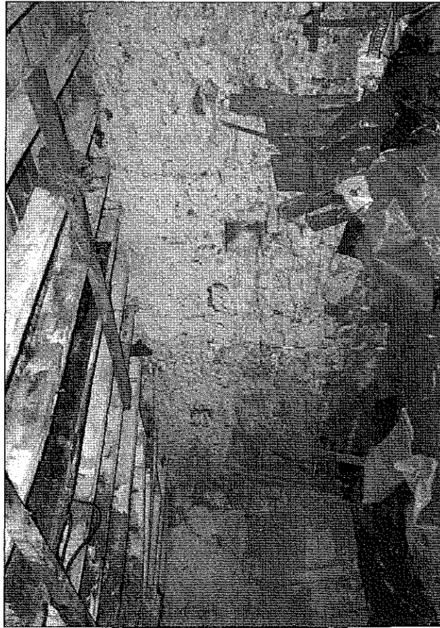
Photo 5: Interior, from the east
