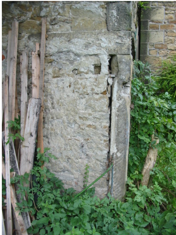
Photo 7 – In-Filled Opening in Gable Wall
