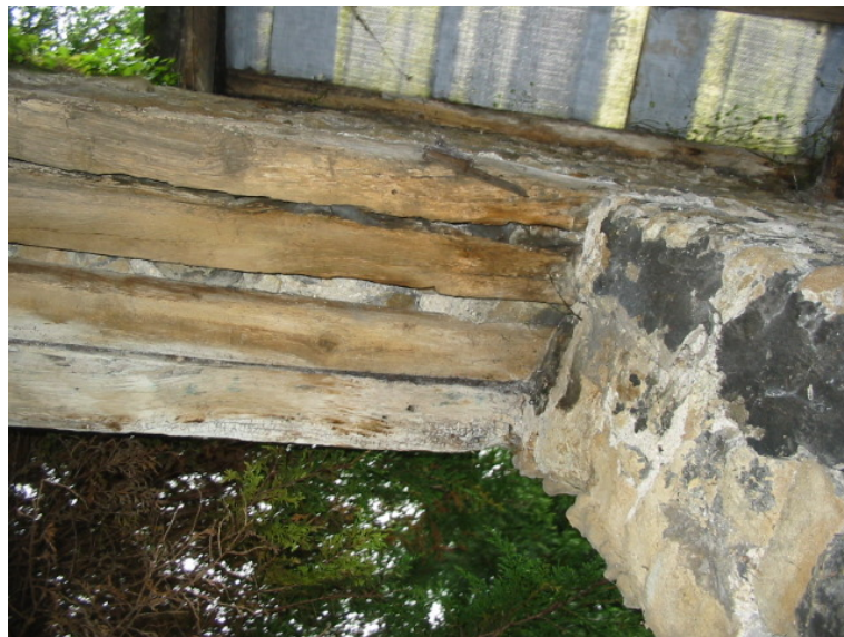
Photo 8 – Decayed Timber Lintels in Gable Wall
