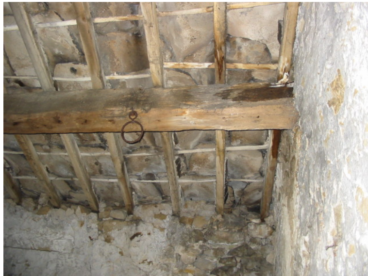
Photo 4 – End of Typical Roof Purlin
