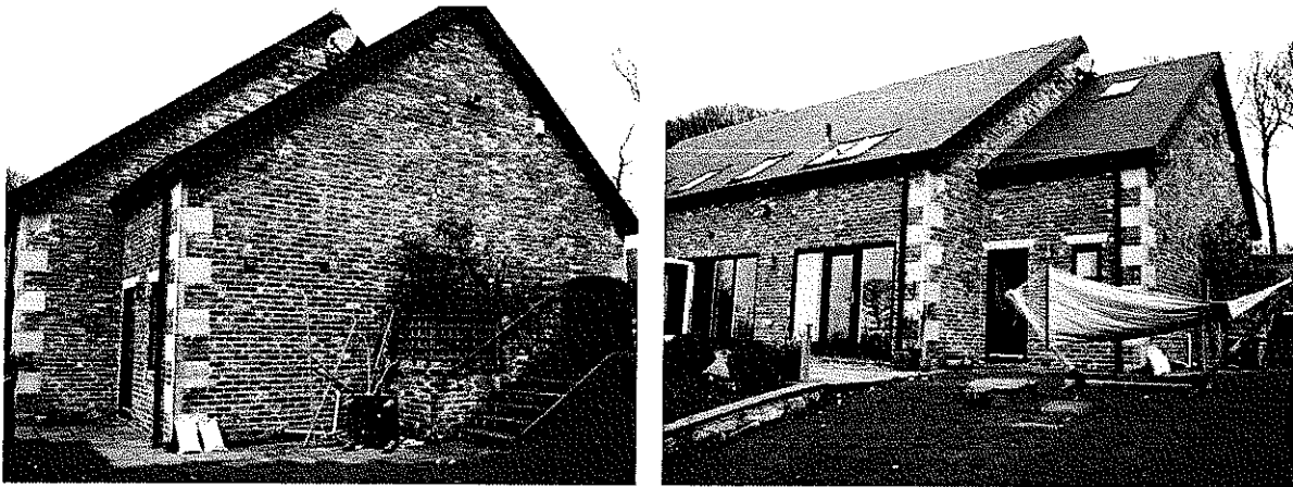
Photographs of part of the East and South Elevation of NO1 the Walled Garden
