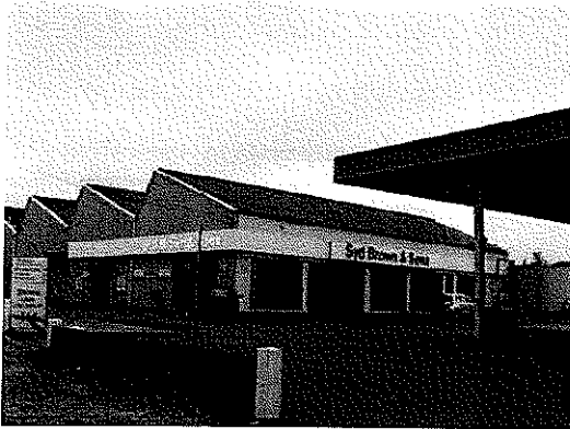
Photo of Syd Brown & Sons garage before Booths refurbishment, taken August 2004
