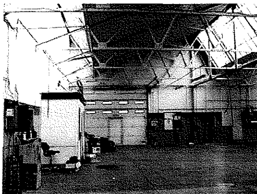
Photo of Syd Brown & Sons garage roof before Booths refurbishment, taken August 2004
