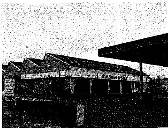
Photo of Syd Brown & Sons garage before Booths refurbishment, taken August 2004
