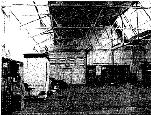
Photo of Syd Brown & Sons garage roof before Booths refurbishment, taken August 2004
