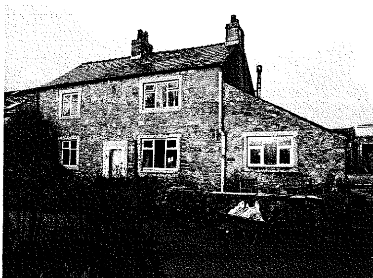
Pl. 2 Photograph showing the South East side of the house
