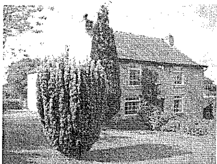
Figure 1: Front (north) elevation
