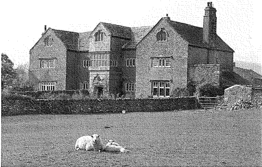
Photo G – Hammerton Hall, Slaidburn
