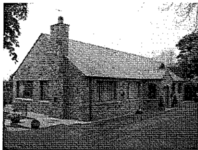
Fig 2: Front (east) elevation.
