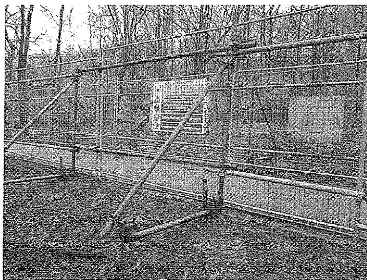
Example of scaffold framework with 'Heras' fencing attached
