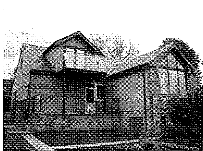
Fig 1: The Eaves (rear elevation)
