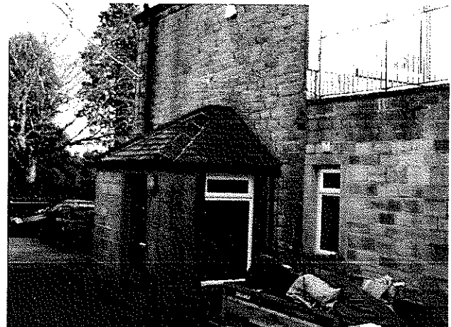
6 North West Elevation to side entry porch
