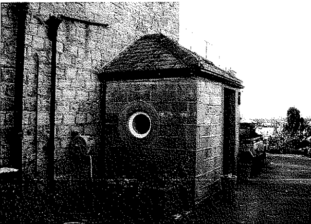
5 View SW to stone side entrance porch
