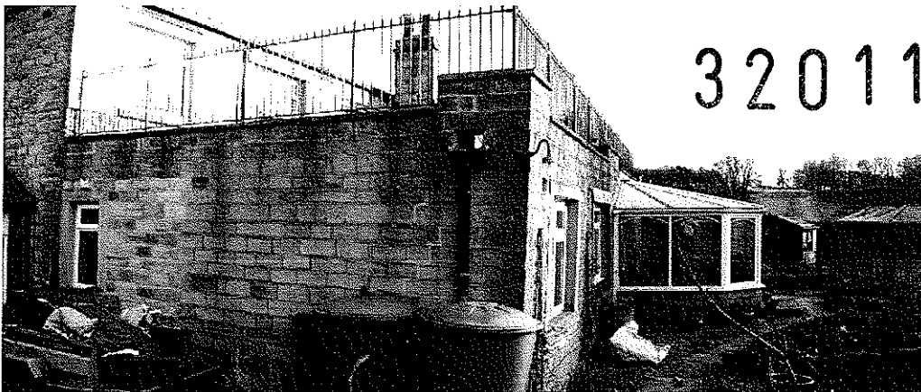
7 View to NW side Flat roof area above is the area for an extension and the conservatory will be replaced
