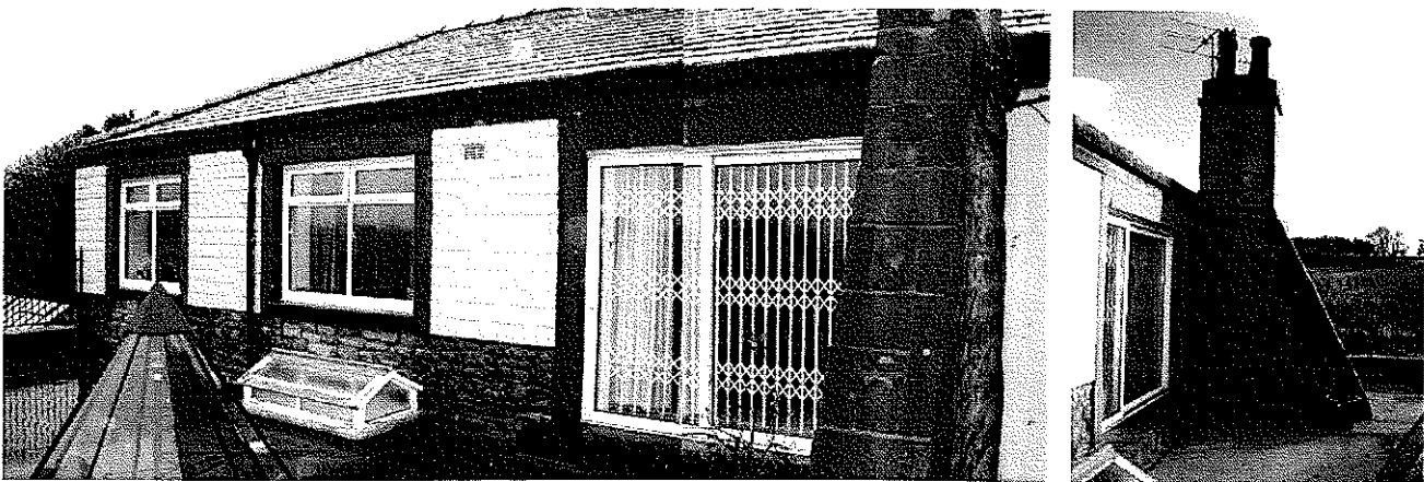
3 and 4 Views across flat roof balcony
