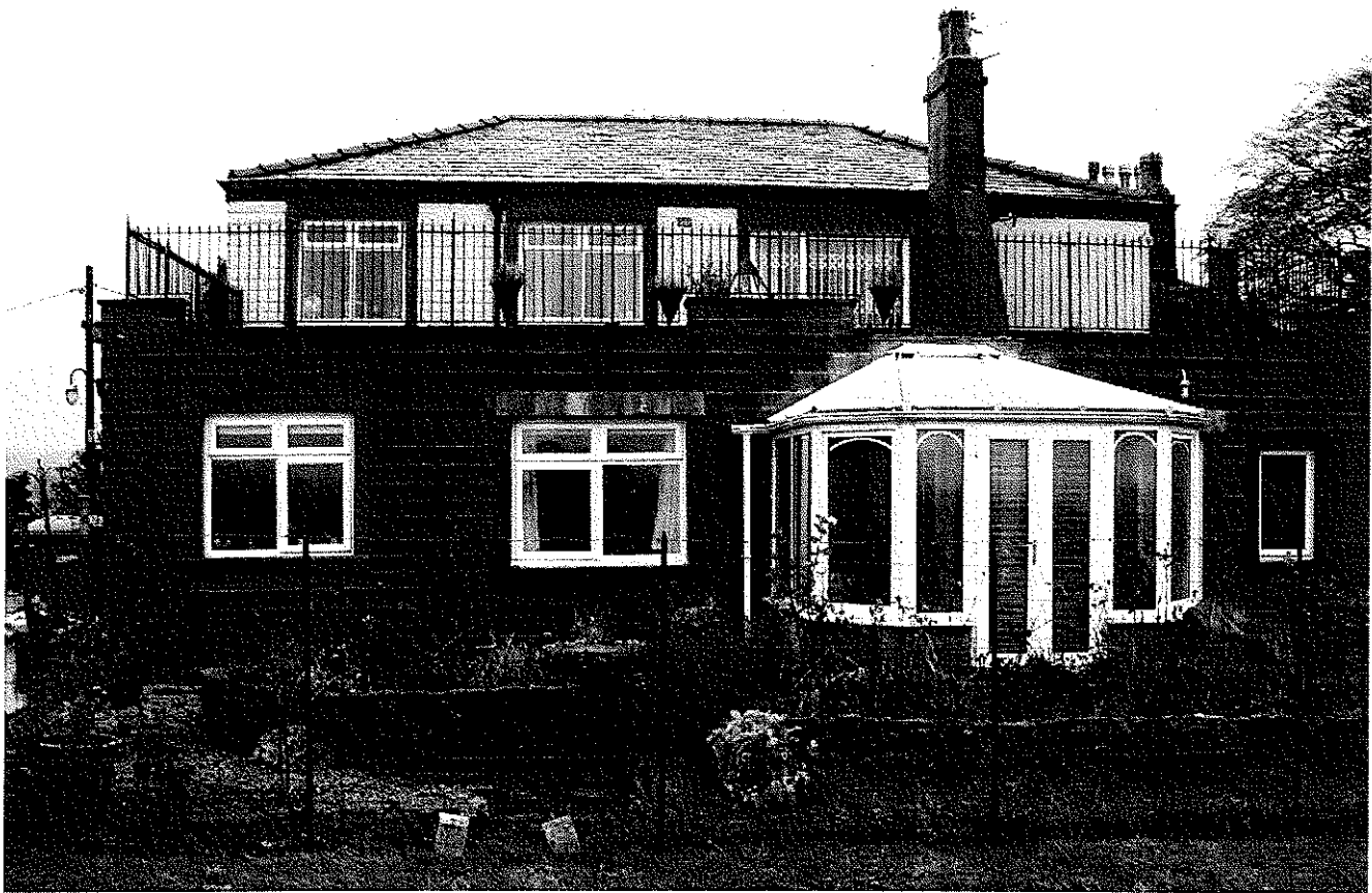
1 Rear South West Elevation showing flat roof and conservatory to be replaced
