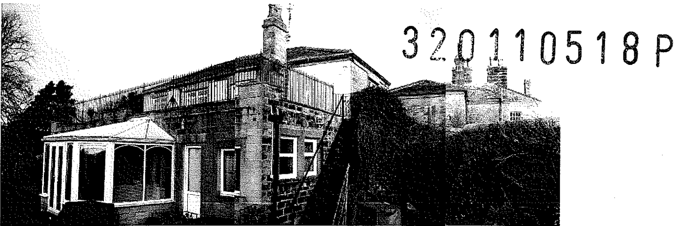
2 View from South to external staircase access and adjacent stone boundary wall
