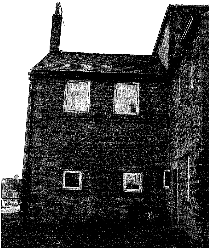
Photograph 32 – Right Side Elevation
