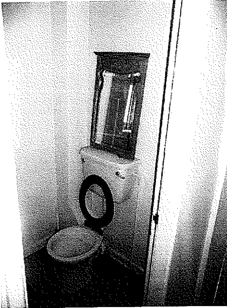
Photograph 9 – Ceramic wc, with existing foul drainage in corner behind boxing
