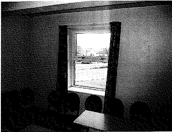
Photograph 15 – Dry-lining to internal face of external wall to left side elevation, uPVC double glazed window
