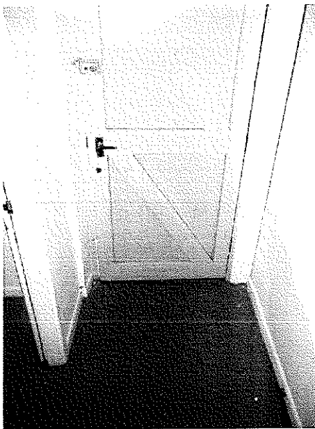
Photograph 8 – Main entrance timber door / sheet vinyl floor finish
