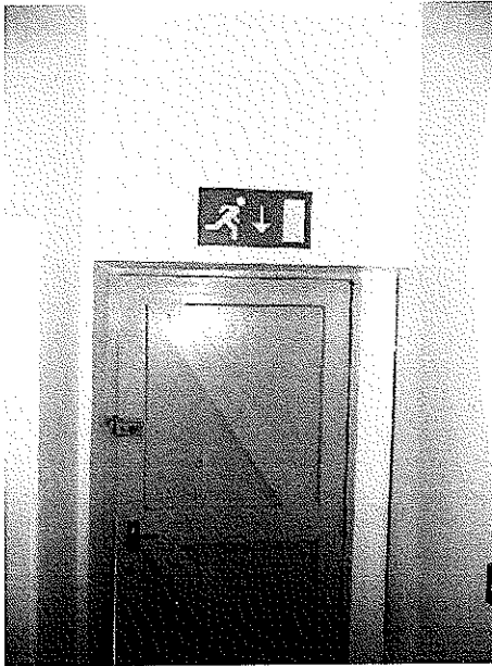
Photograph 7 – Internal face of external wall to front elevation
