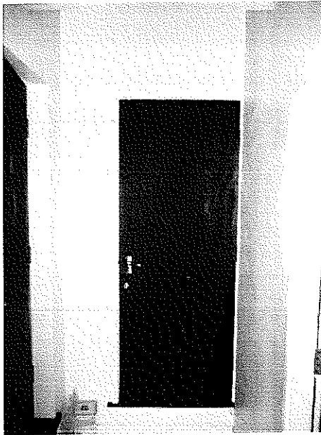
Photograph 4 – Modern timber door to cupboard
