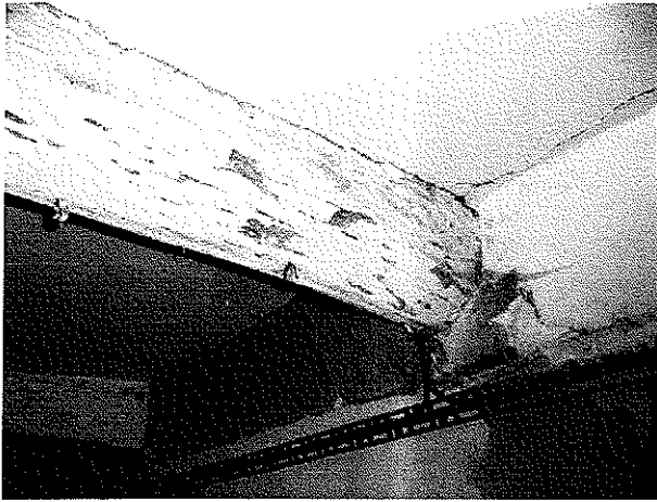
Photograph 27 – Existing original timber floor joist
