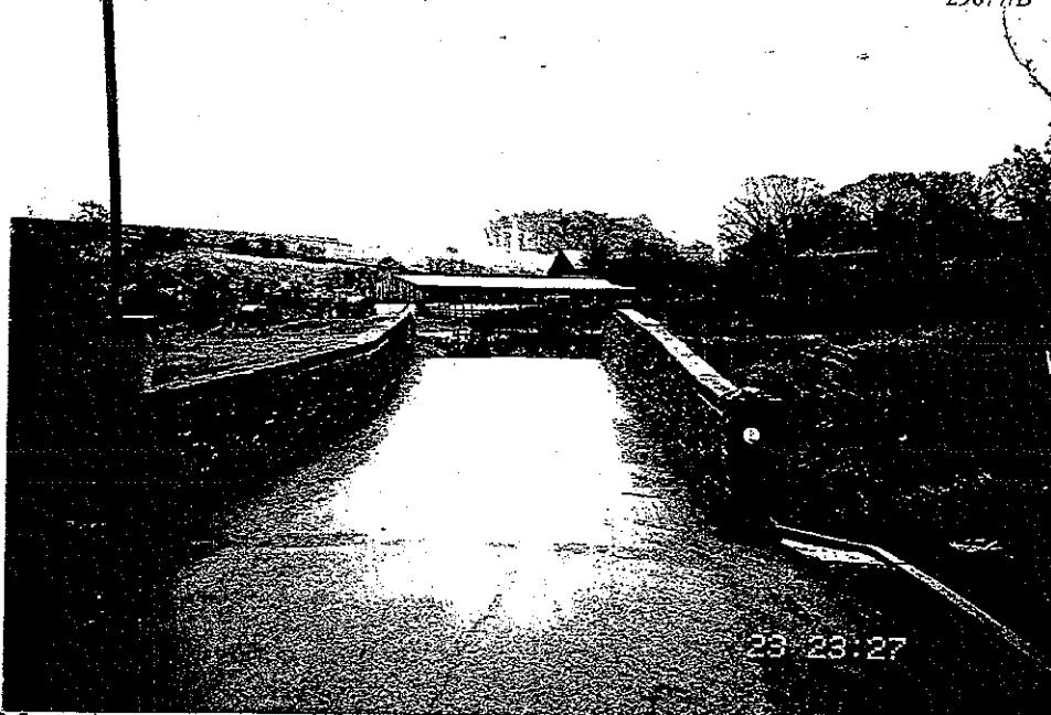
3.2 APPROACH FROM THE NORTH
