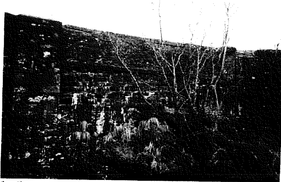
P13 GENERAL VIEW OF SOUTH WEST WINGWALL
