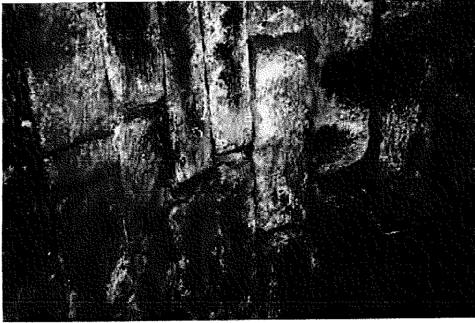
P20 RELIEF ARCH - OPEN JOINTS 29677/3/16
