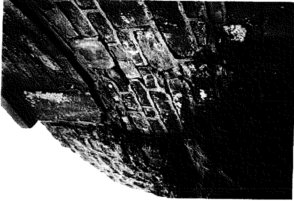
P16 S.E. WINGWALL - REPOINTING/MOVEMENT
