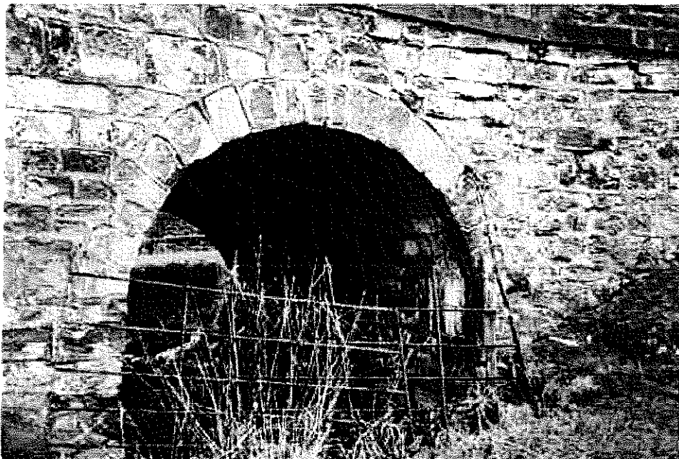
P24 EAST ELEVATION OF RELIEF ARCH
