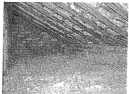
Figure 3: Roof void (eaves at front)
