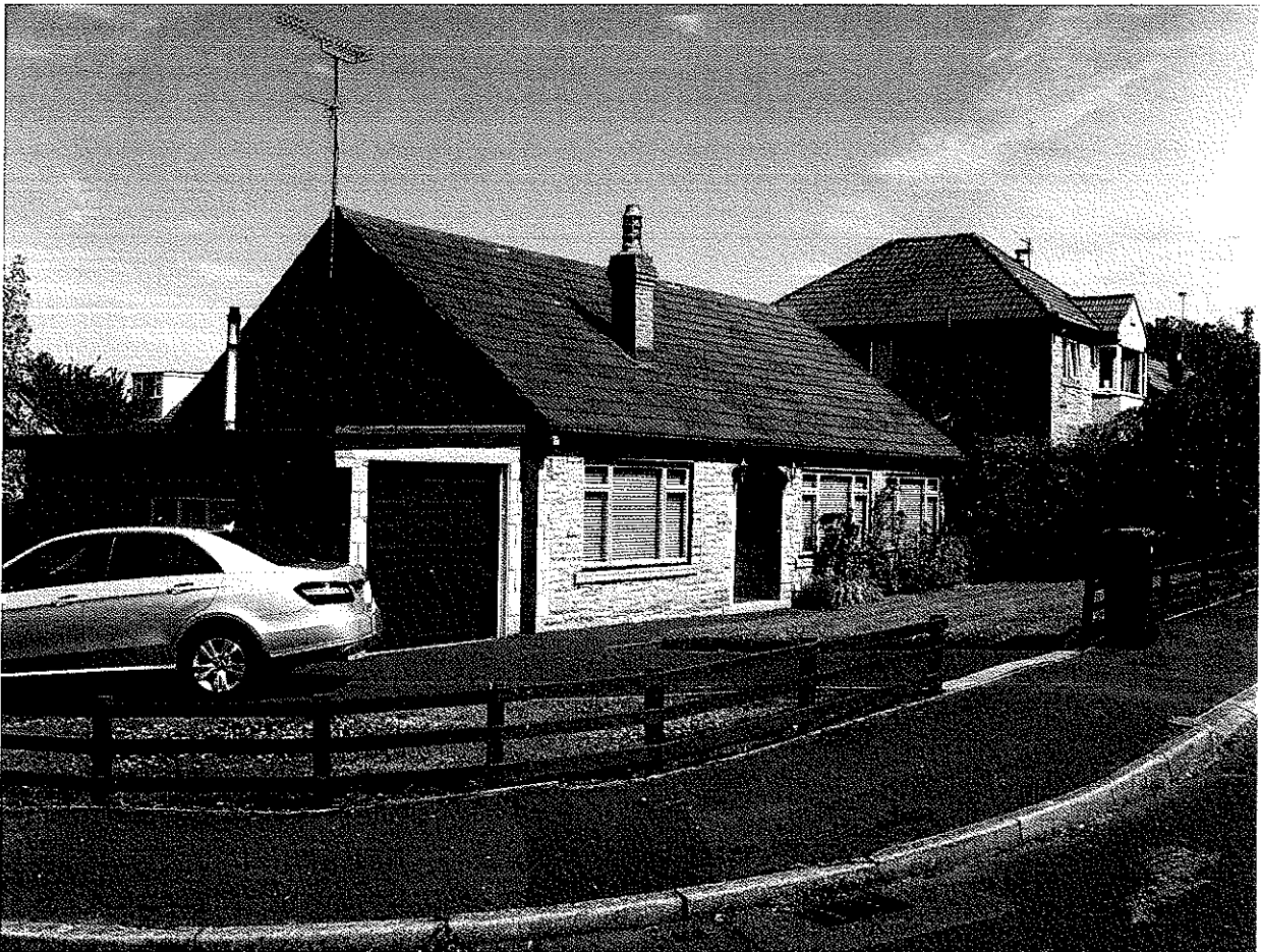
View of 24 Chatburn Park Drive Front Elevation from the South
