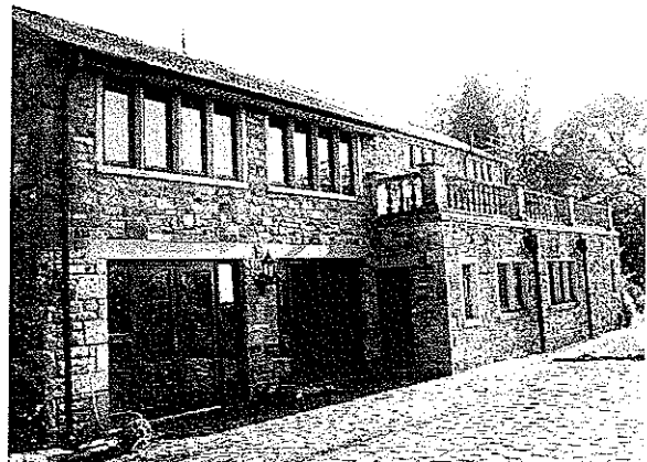
North elevation patio doors and rear door.
