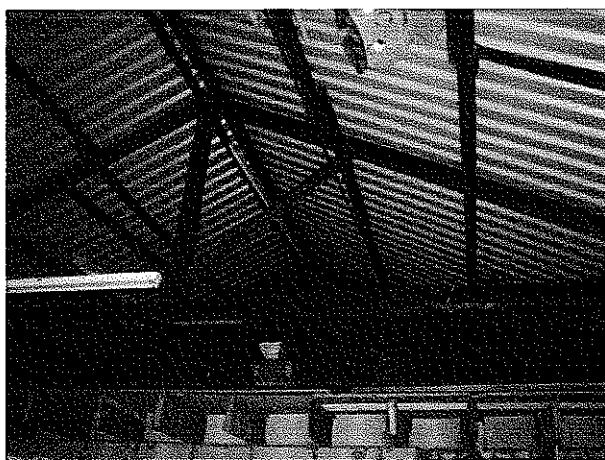
Internal view of Garage/store roof.
