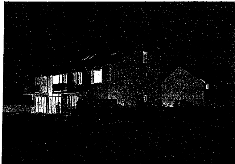
2: Rear Elevation by Night
