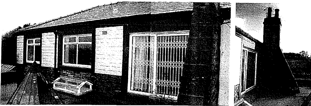
3 and 4 Views across flat roof balcony
