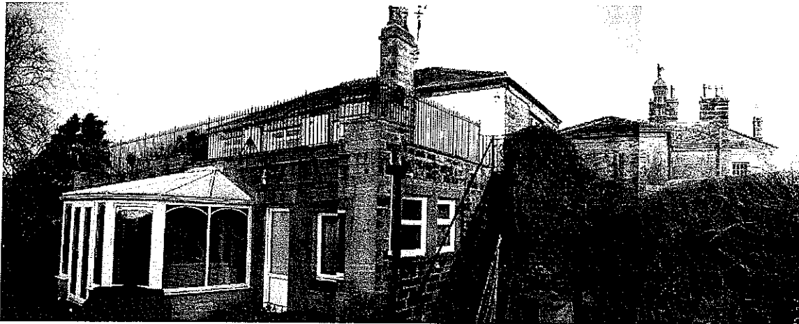
2 View from South to external staircase access and adjacent stone boundary wall
