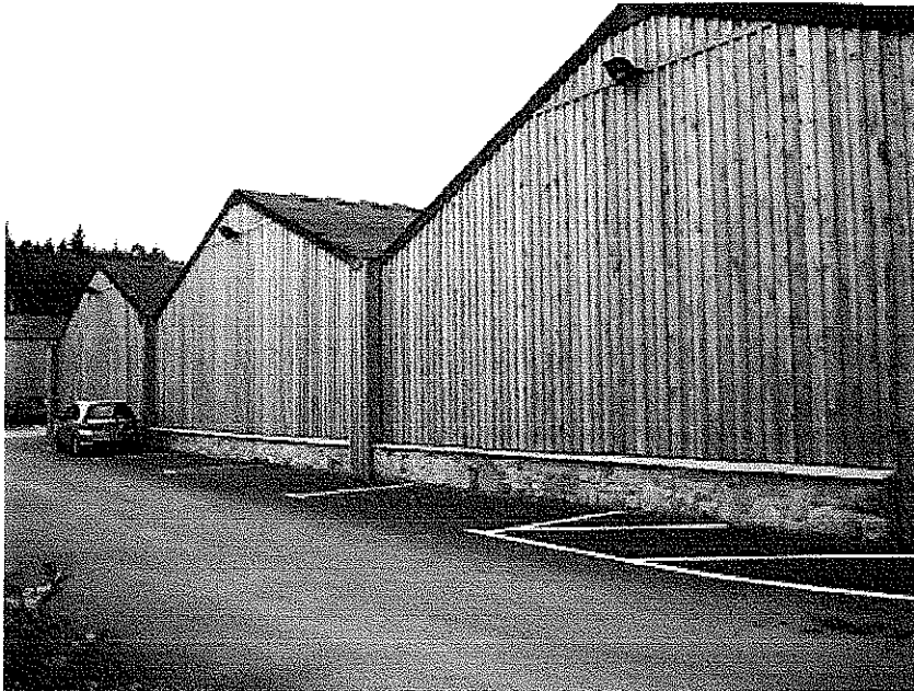
Barn No 5 – North East elevation where the office entrances will be located.
