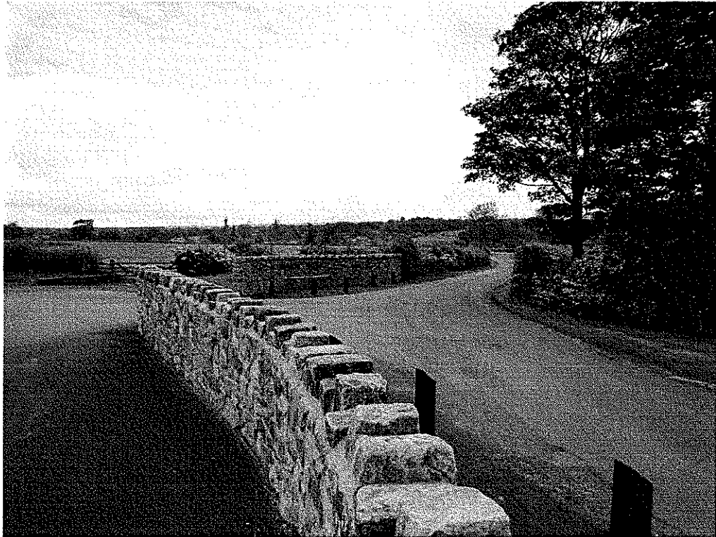
Recently improved access to serve both phase 1 & 2
