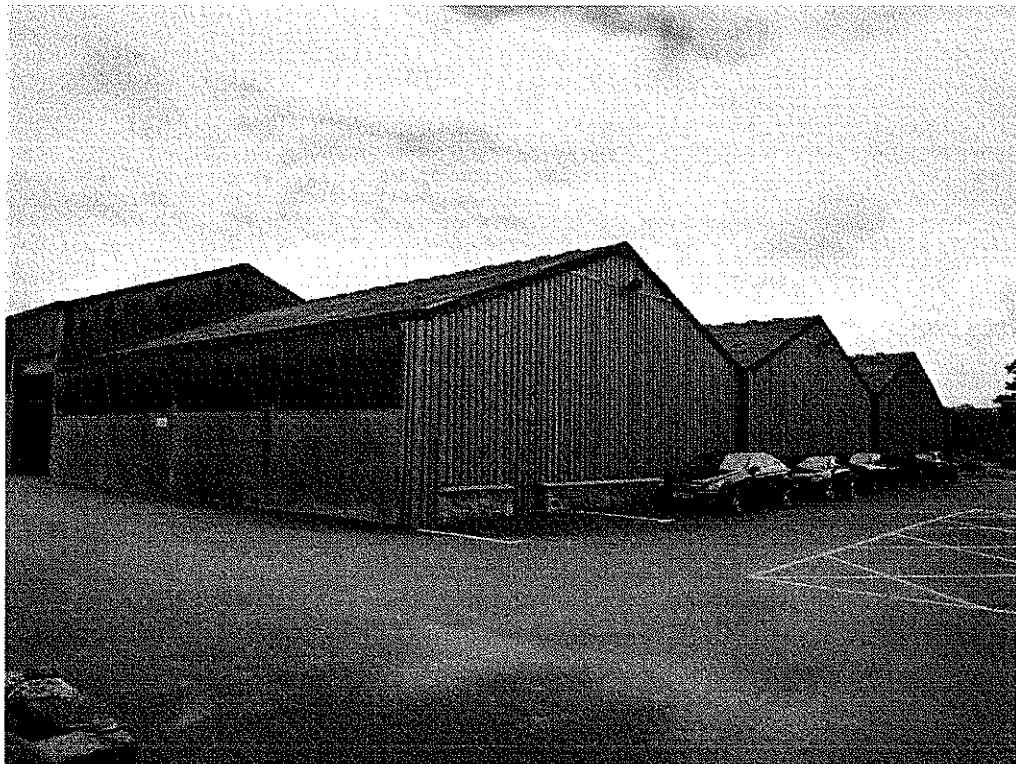
Former agricultural building to be partly converted to B1 use
