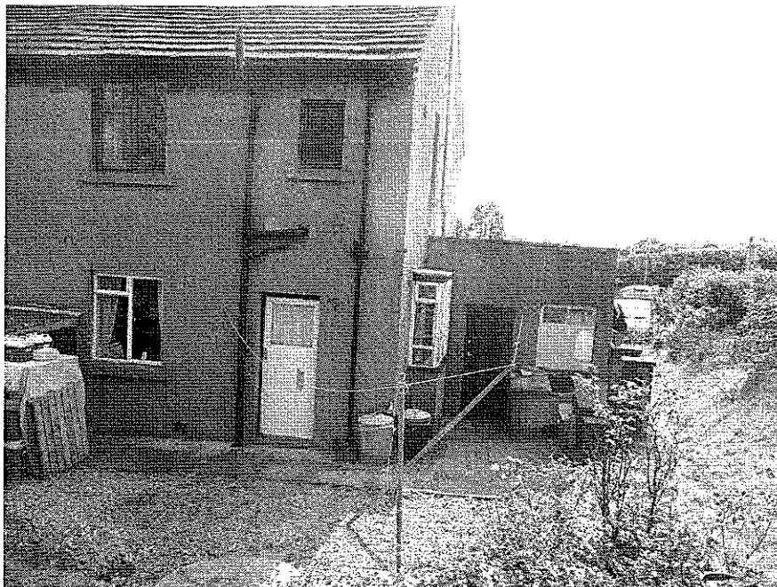
Rear elevation and view of the site of the
