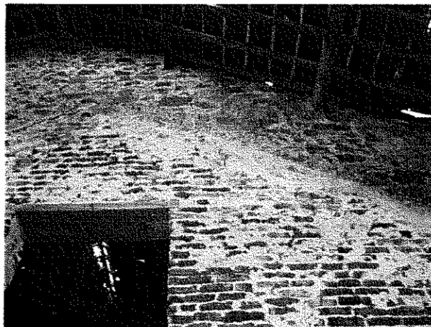
36. Evidence of former structure noted by the outline of pitched roof
