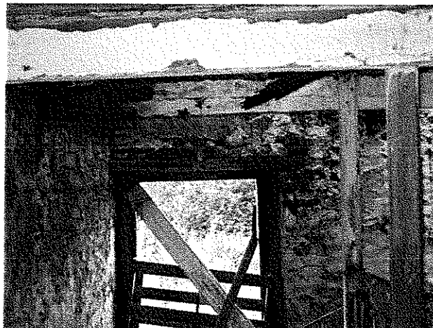
33. Timber lintel to opening on external wall
