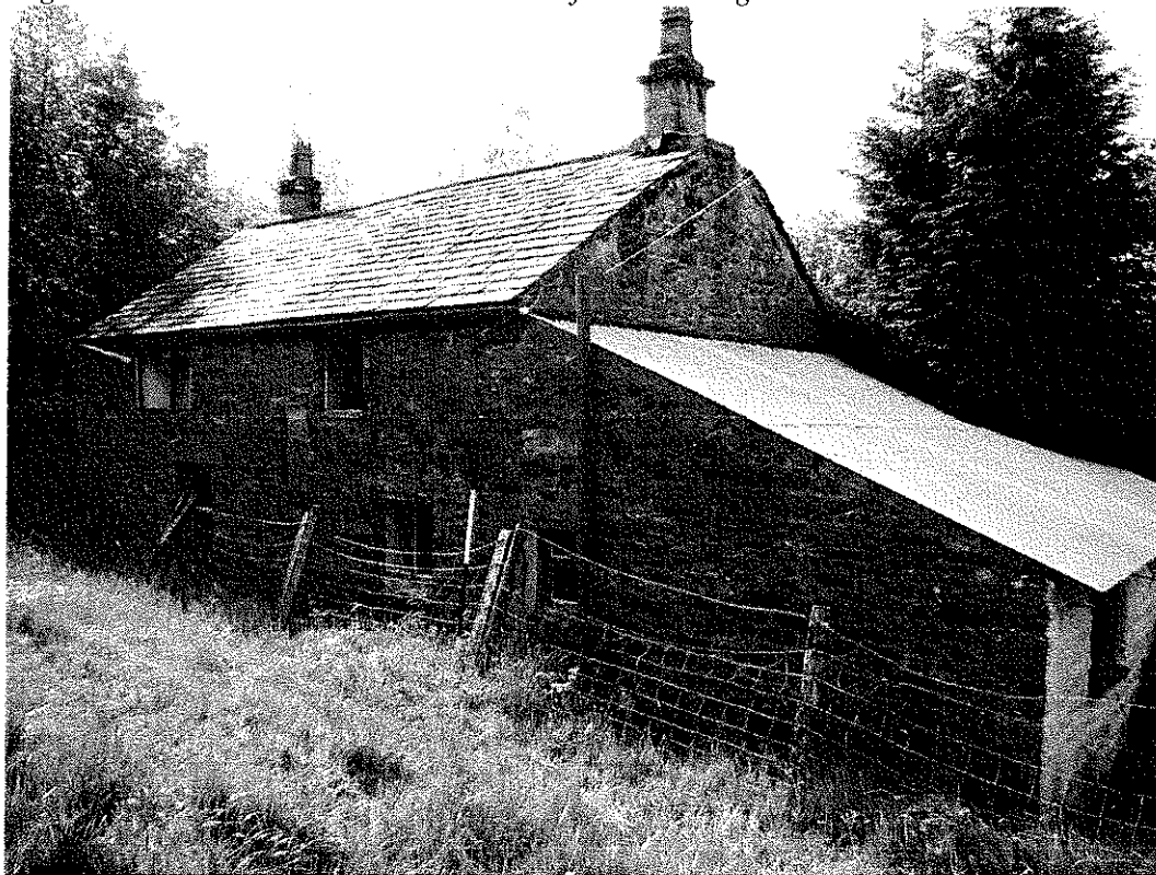
4. Southern elevation facing pasture the sloping nature of the ground can be seen. The eastern lean-to is at the right of the shot with the main two-storey section of the building central
