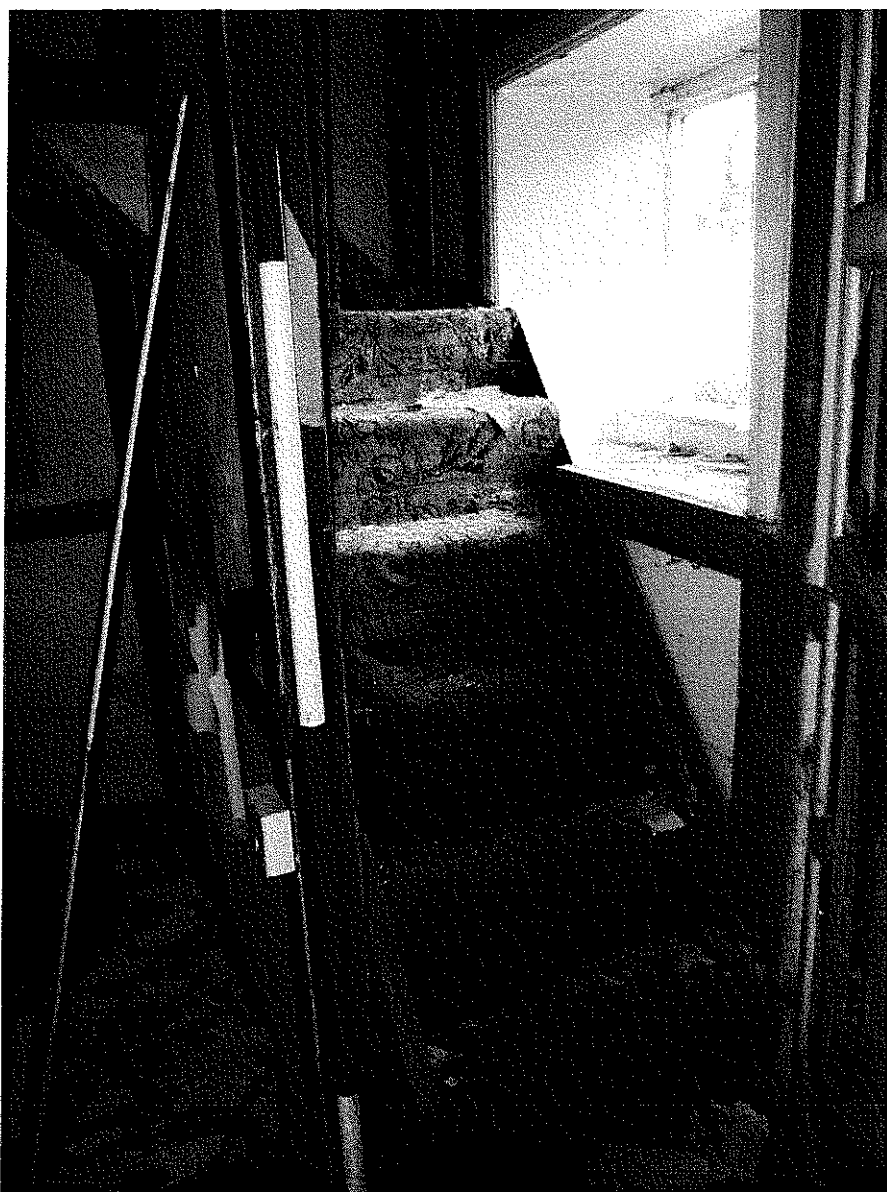
20. The staircase from the eastern ground floor room (of two storey part). That this cuts partly across the window is another indicator that it was inserted
