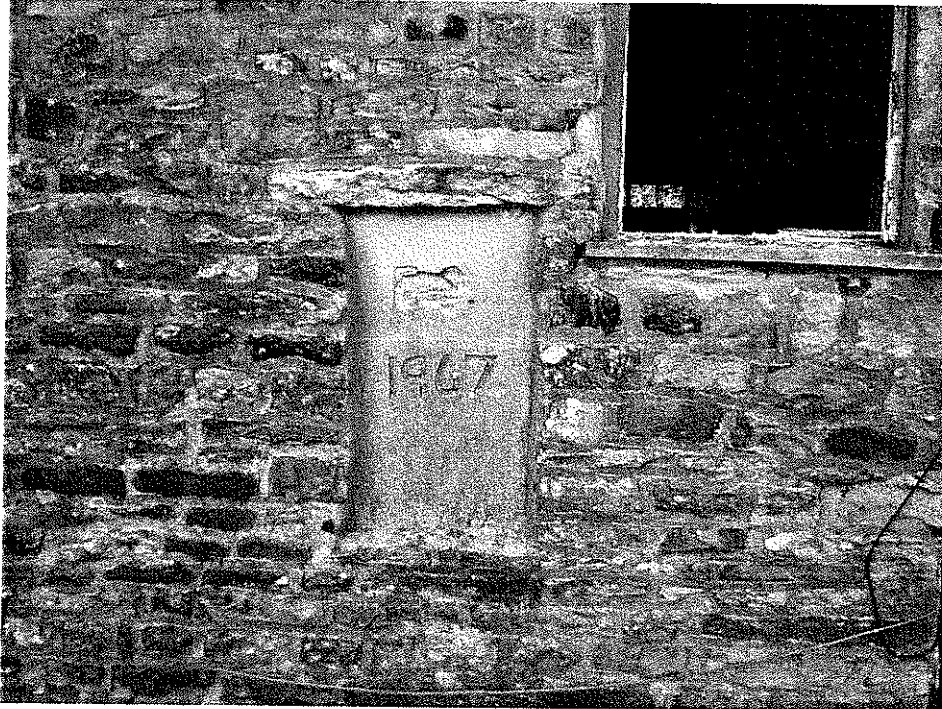
6a. Cemented datestone to southern elevation inserted in possible previous window opening. Quite what the 1967 commemorates is unclear, but it is possible that the cottage may have been renovated at this time
