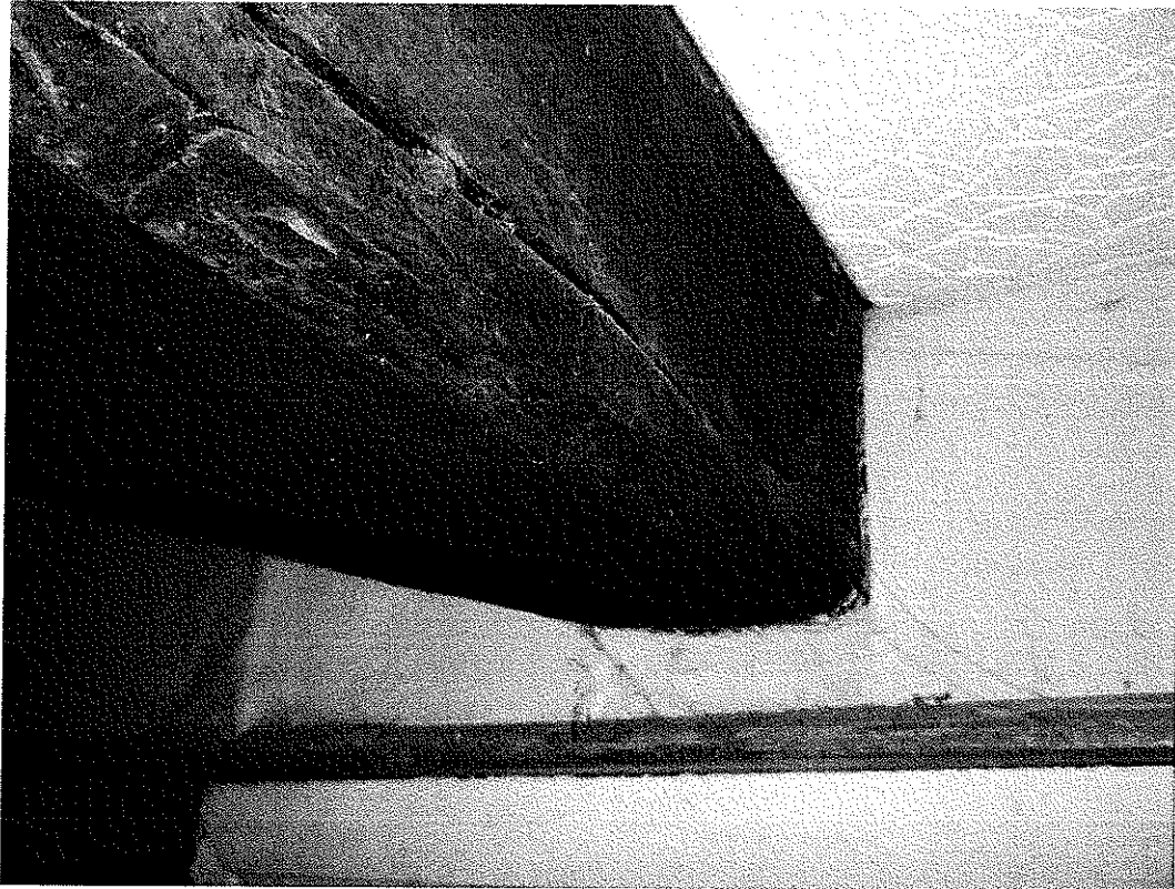
24. As 23, showing chamfer to beams (without stops)
