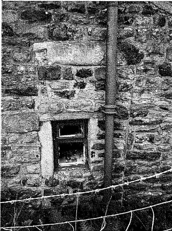
6c Southern elevation, window in former door opening to eastern lean-to
