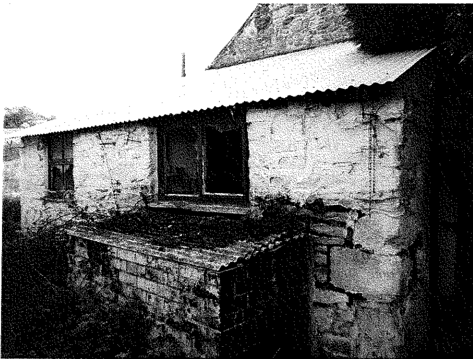
3. Eastern lean-to addition of rubble construction with a sheet covered rafter roof. An entry door to the north wall of this addition can be seen to right beneath the heavy vegetation that surrounds the north side of the building
