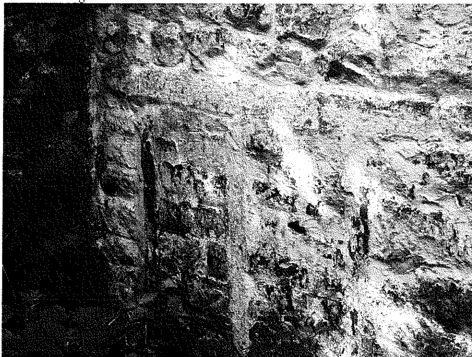
11. Blocked twin light mullion window to the western gable at ground floor level. This former window was probably blocked when the lean-to to the west (only part remaining) was constructed. The square mullion profile (to the face) is indicative of C18th construction.
