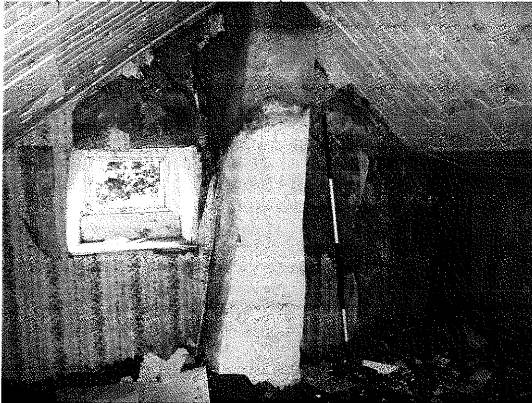
15. First floor western room chimney flue to western gable serving fireplace to ground floor below
