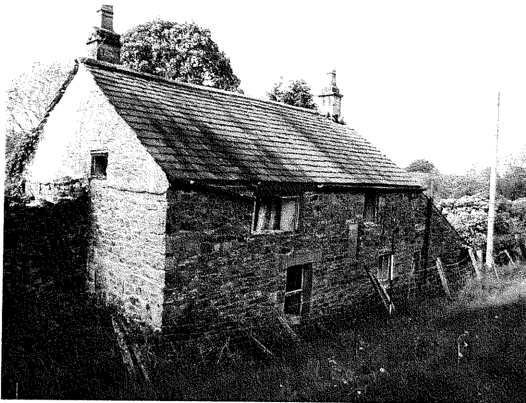
9. View from the south west showing small gable window inserted over the line of what appears to have been a full gable width lean-to structure.
