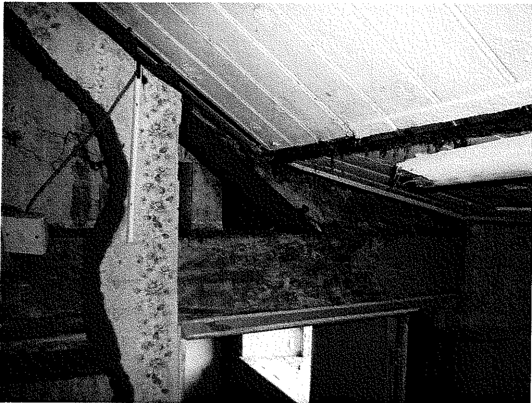
13. As 12, doorway with low head (1.2m) through to adjacent room formed by cutting out lower edge of truss tie. Here the cranked profile of the principal can also be seen where the principal meets the tie. The alteration of the tie beam and low head of the doorway here suggests that connection between the two upper rooms was an insertion rather than an original feature. This in turn indicates that the cottage was either a) at some stage two separate adjoined dwellings or b) a single storey (open to the roof) dwelling into which the first floor was added (see also later).
