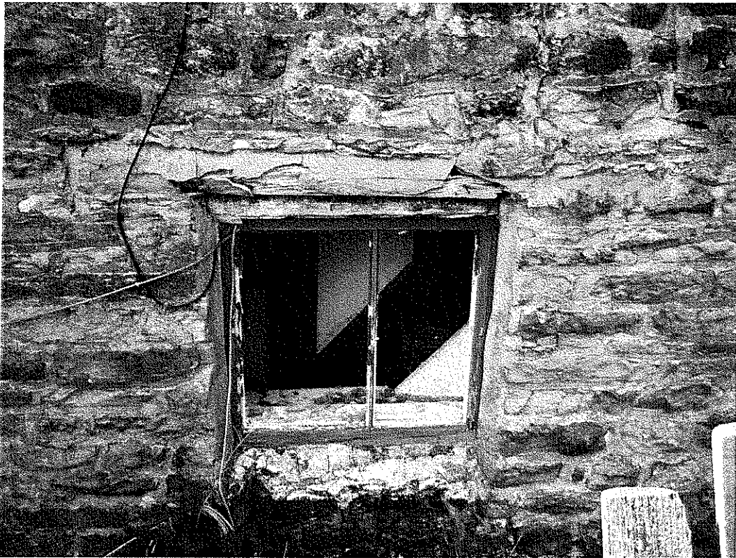
6b. Inserted window to southern elevation, ground floor to right side of two storey part, with cement covered timber lintel.
