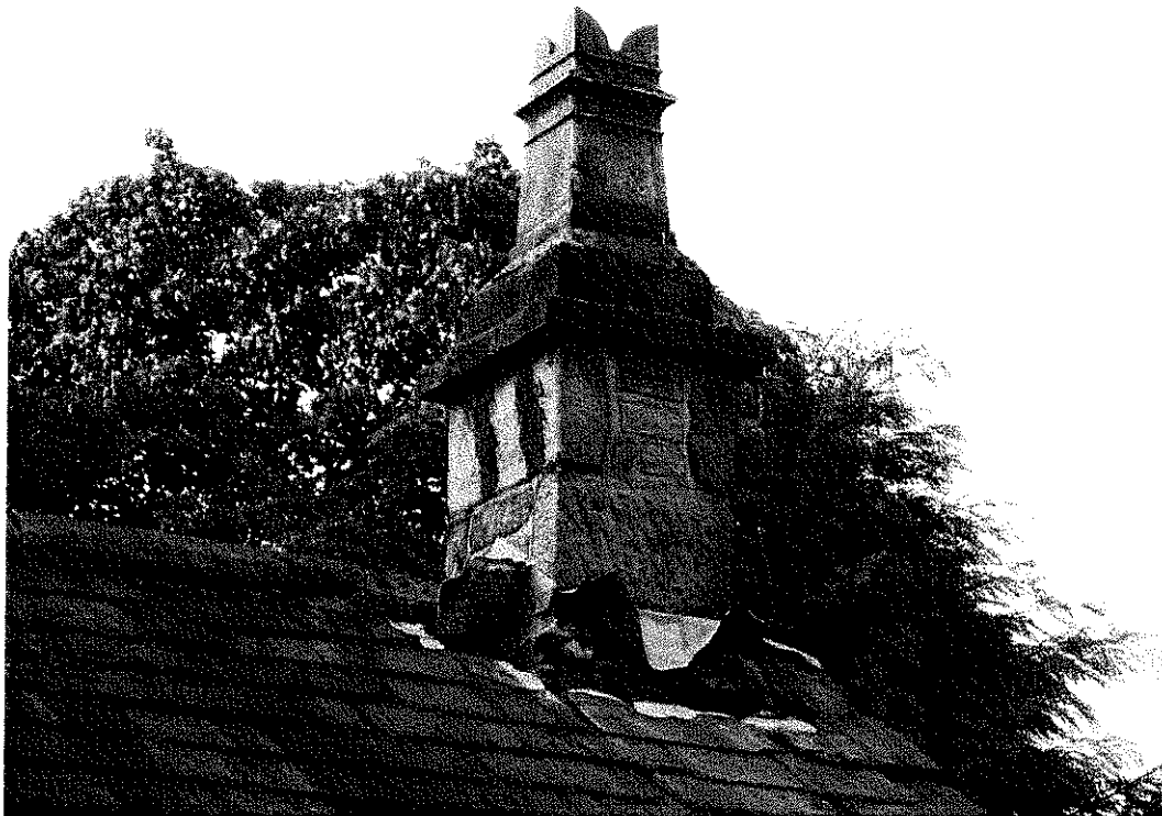
7. Eastern chimney (single flue)
