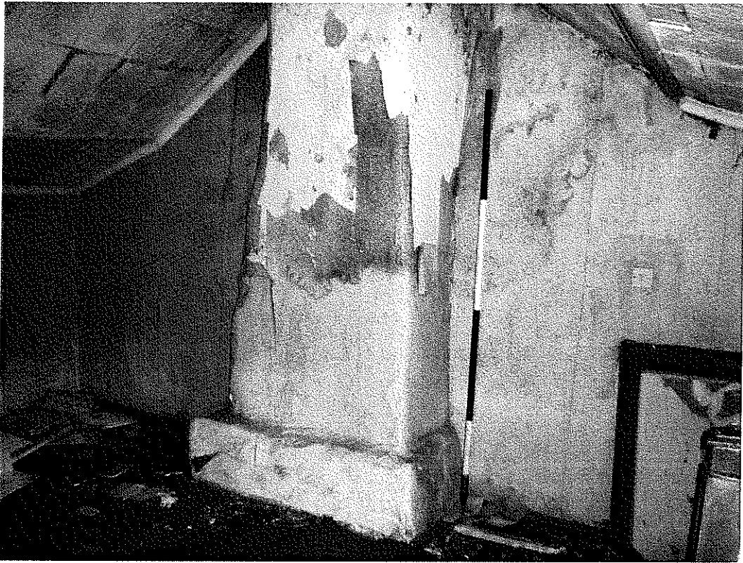
16. Eastern first floor room, single flue to eastern gable The cranked profile of the ceiling can also be seen indicating the unusual nature of the roof structure above
