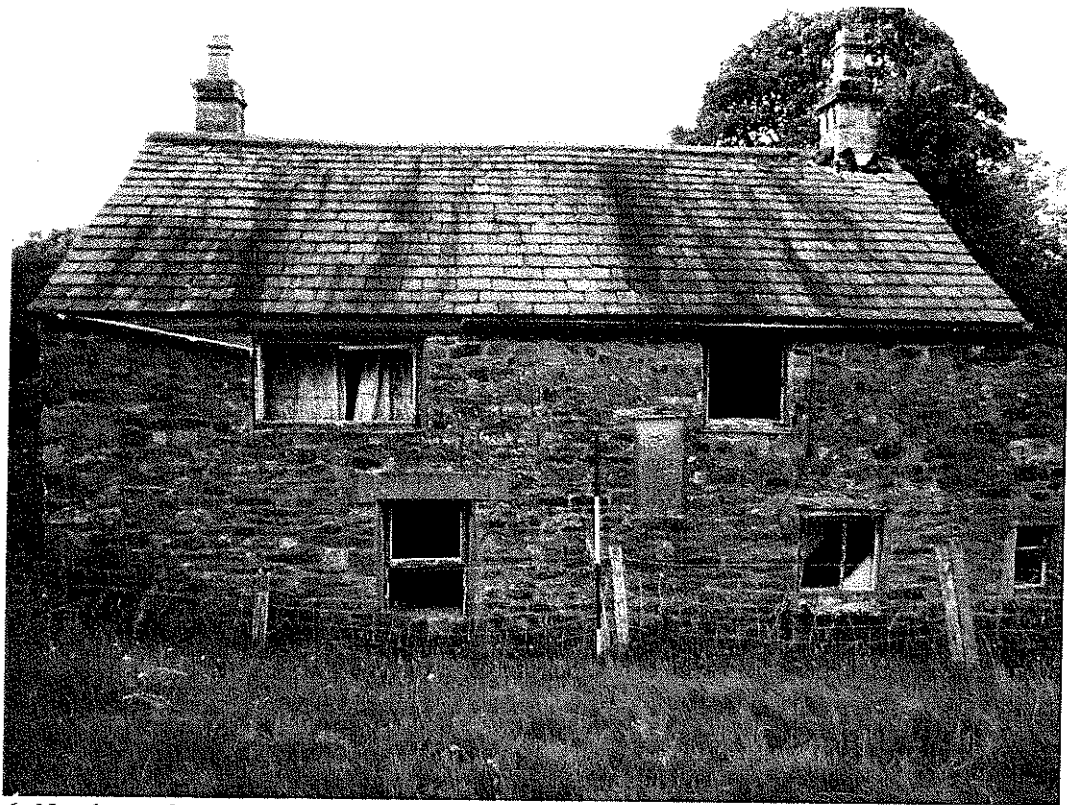
6. Northern elevation, main two storey part. The upper left window appears to have been widened, whereas the lower inner right window is inserted
