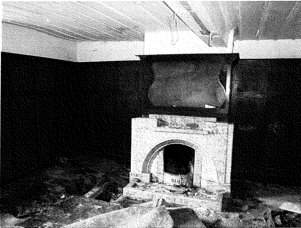
25 Western ground floor room with chimney to west gable The fireplace is probably C20th as is the wall panelling. Only a single central beam is evident. This differs from the adjacent room where two beams are present.
