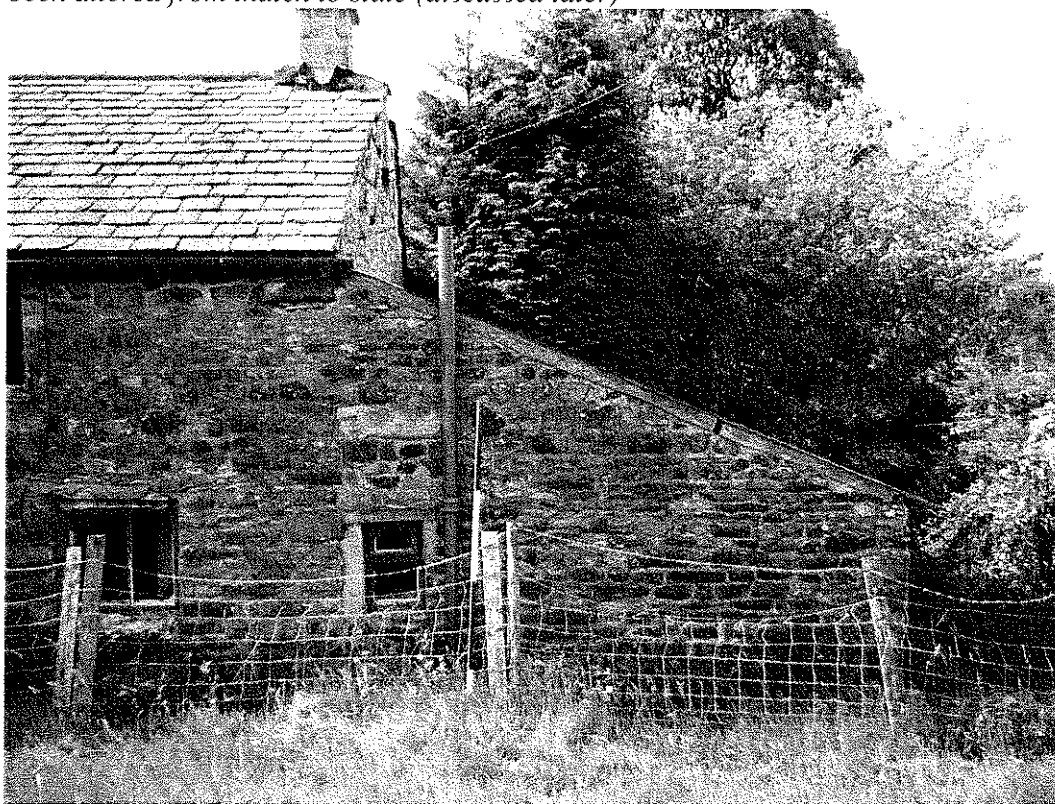
5 Southern elevation with eastern lean-to junction to main two storey part. Here original quoins of the two storey part have been swung around to provide a starting 'key' for the lean-to addition.
