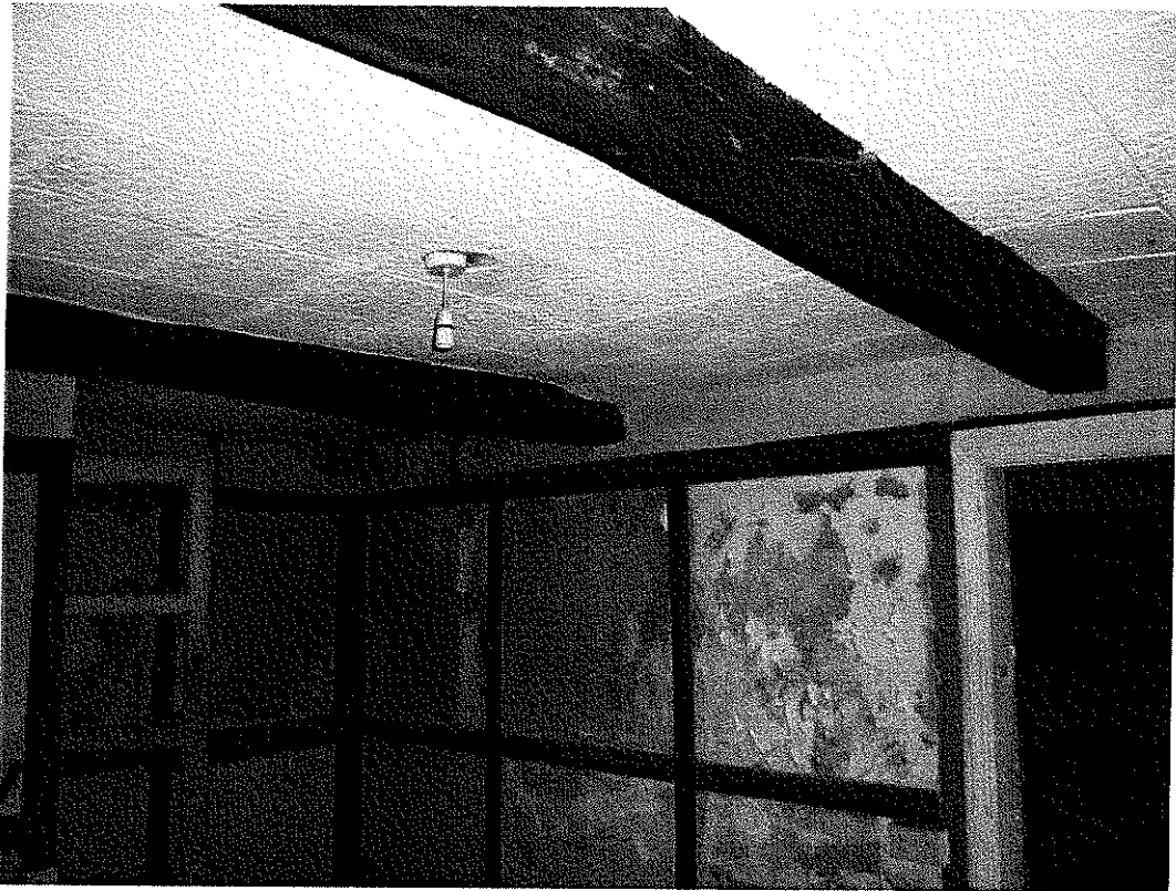
23 First floor beams over eastern ground floor room. The wooden wall framing is applied rather than structural
