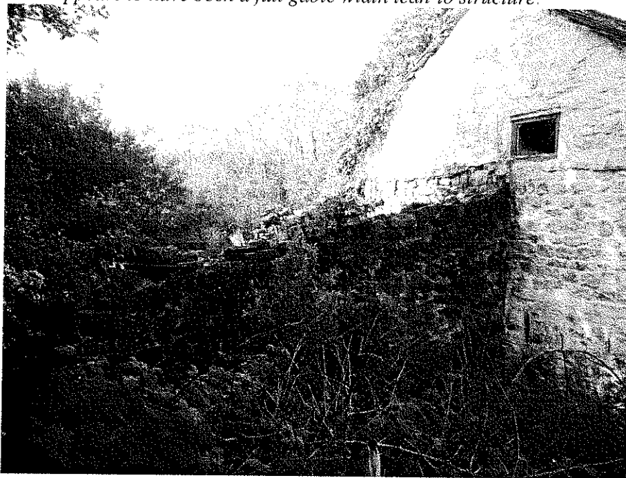
9a. Reduced dilapidated lean-to against the western gable The photo also shows thick undergrowth against the north and west of the building which prevented inspection of these parts externally
