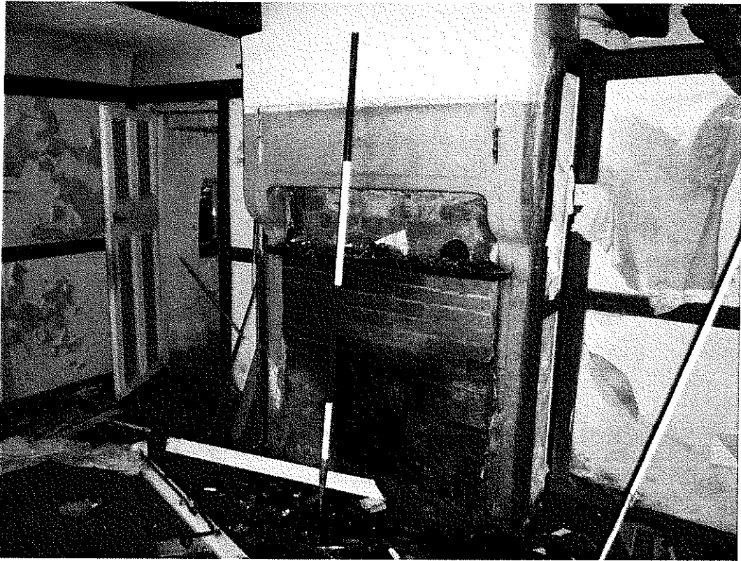
21. Eastern ground floor room of two storey part. Fireplace to eastern wall with stone chimney piece and corbelled mantelshelf. This is likely to be C18th. Two first floor beams can be seen to the left and right sides of the chimney
