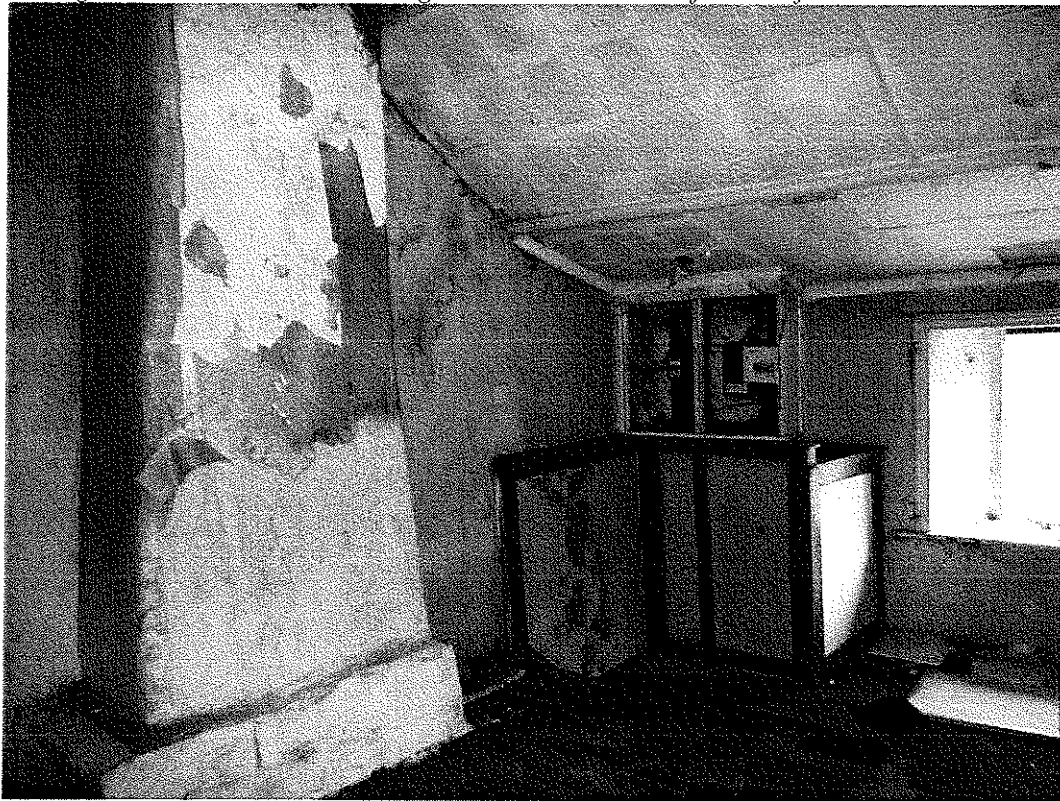
17. Eastern first floor room, looking to stair in south east corner
