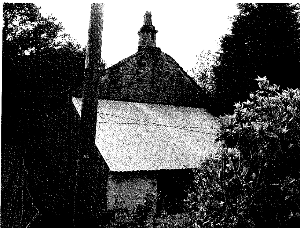
4a Eastern gable over the lean-to The irregular nature of the stonework at high level indicates past alteration work, possibly building up when the roof covering may have been altered from thatch to slate (discussed later)
