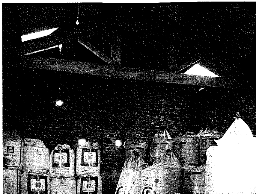
Photo 8 – Traditional roof truss
