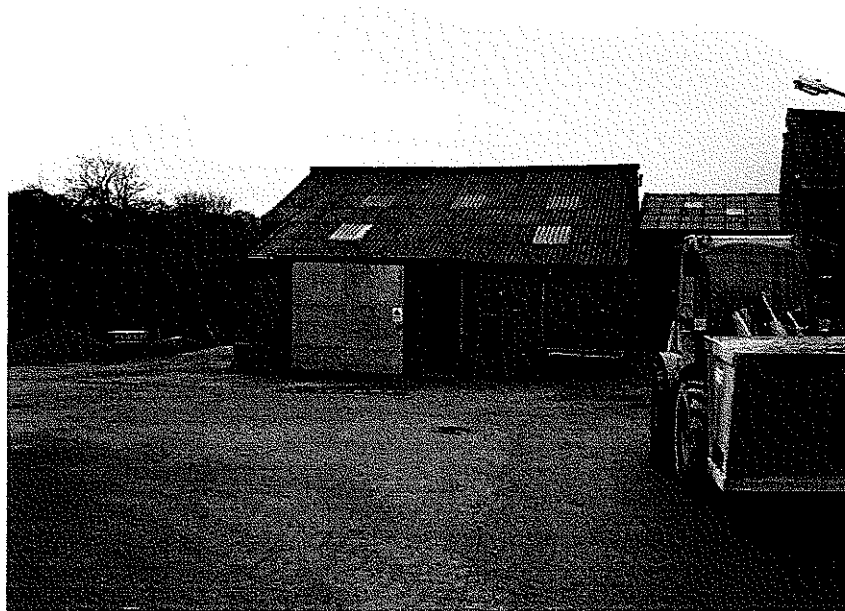
Photo 3 – Existing West Elevation
