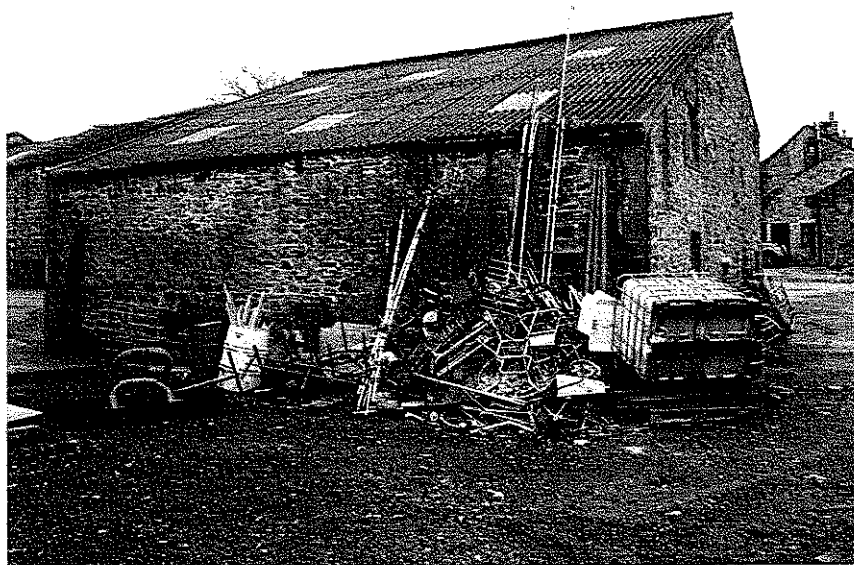
Photo 5 – Existing East Elevation (Lean-to)
