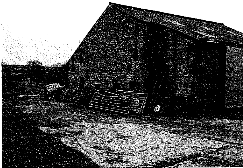
Photo 4 – Existing North Elevation
