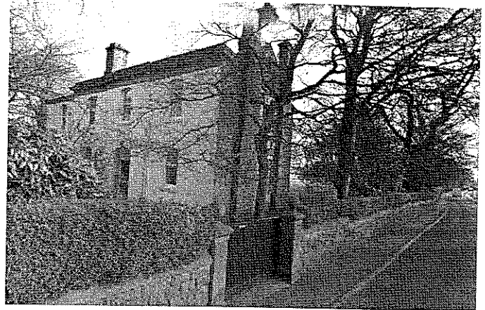
Fig 33. Dilworth House West elevation
