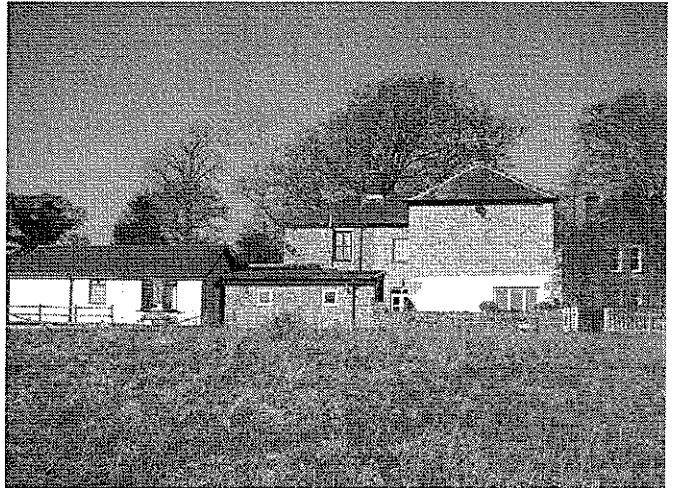
Fig 5. South elevation 39 (left) & 41 Dilworth Lane
