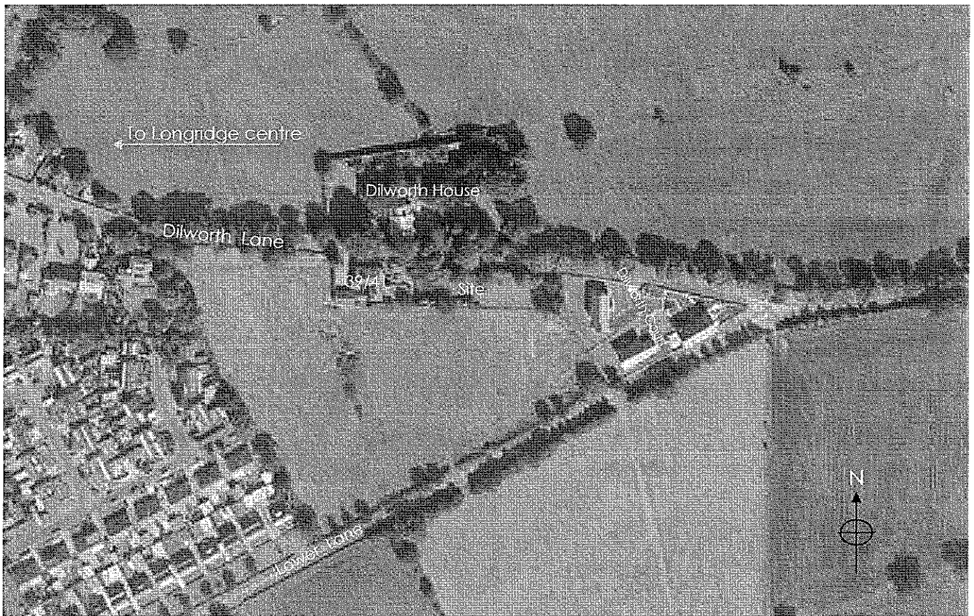
Fig 1. 39+41 Dilworth lane. Aerial view of site.
