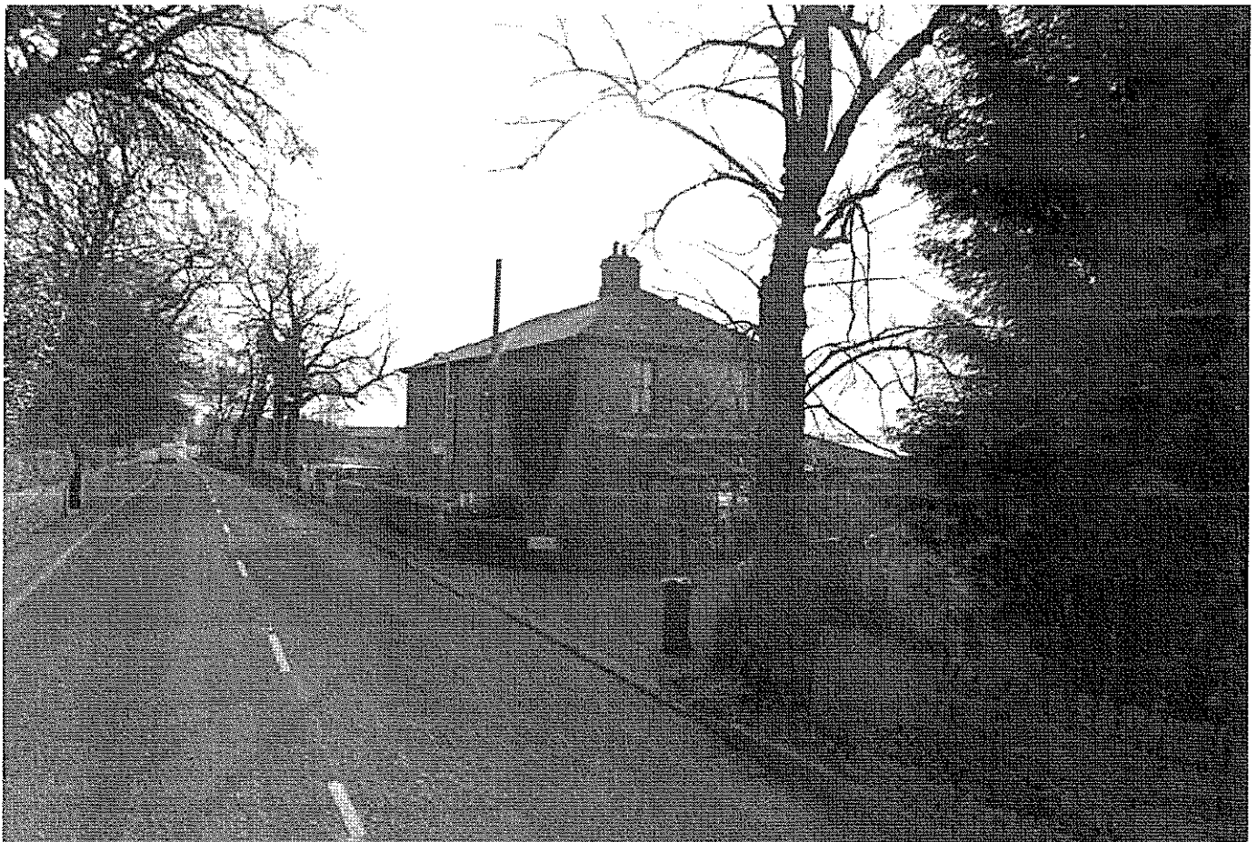
Fig. 36 Same elevation , as seen today depicts the large conservatory addition.
