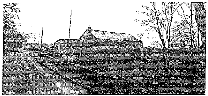
Fig 3. Dilworth Court Housing to the East of the site
