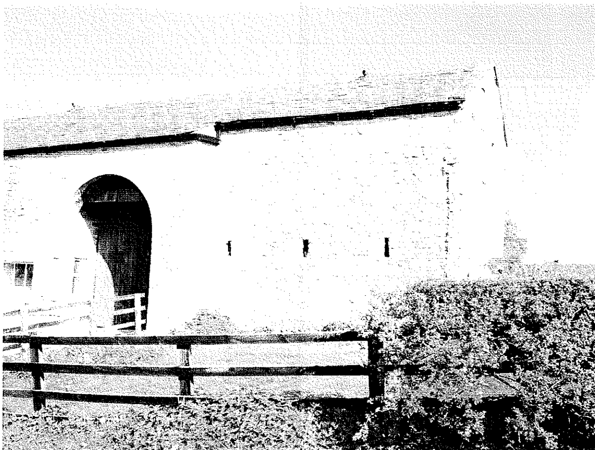
Image 2: Front side of the barn showing interesting features such as the three ventilation slots
