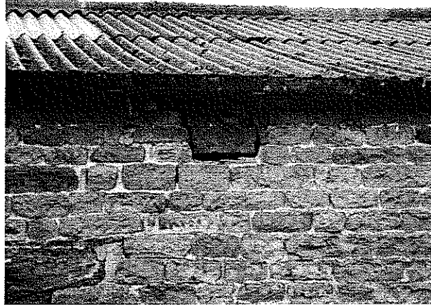
8. Arched timber lintel above cart opening to barn 2
