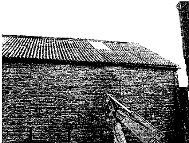
12. Westerly gable wall of barn 2 and side wall of lean-to
