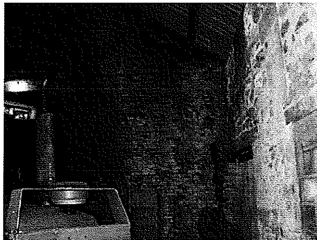
29. Cracking at join between stone and brick work sections of separating wall
