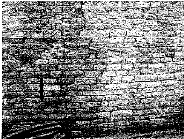
9. Re-pointed section of wall to front wall of barn 2, that has suffered structural movement
