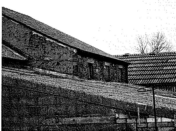
17. Poor flashing detail of barn 2 roof to separating wall. Defective render to wall of barn 1
