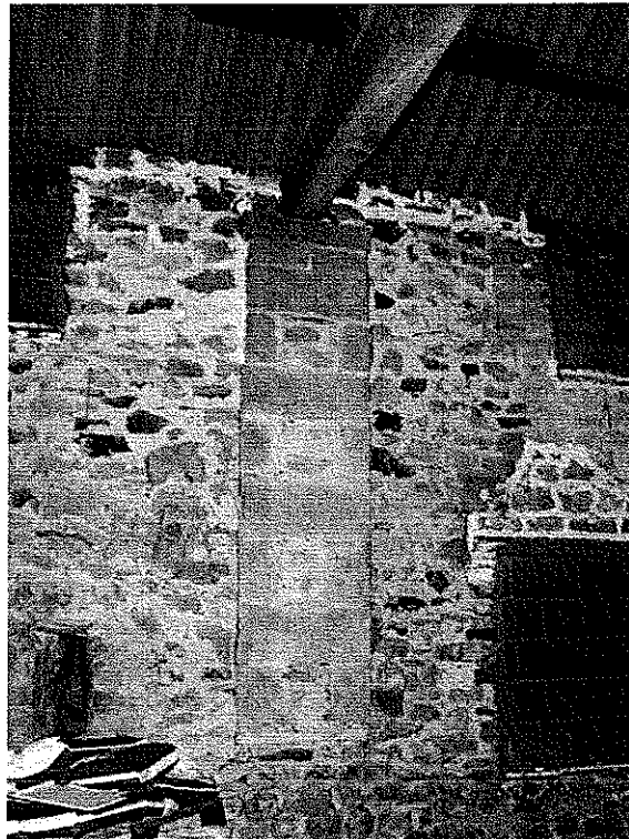
34. Roof trusses sat on stone piers to rear wall within barn 2
