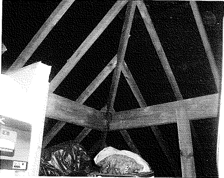
ROOF SPACE MAIN ROOF
