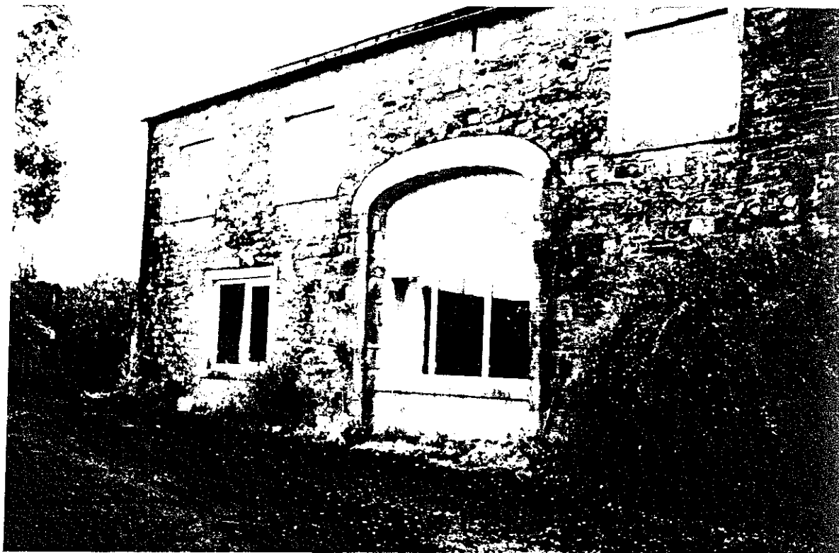
REDHILL GATE BARN BULTON E./BOWLAND Multiple new windows to east and south front
