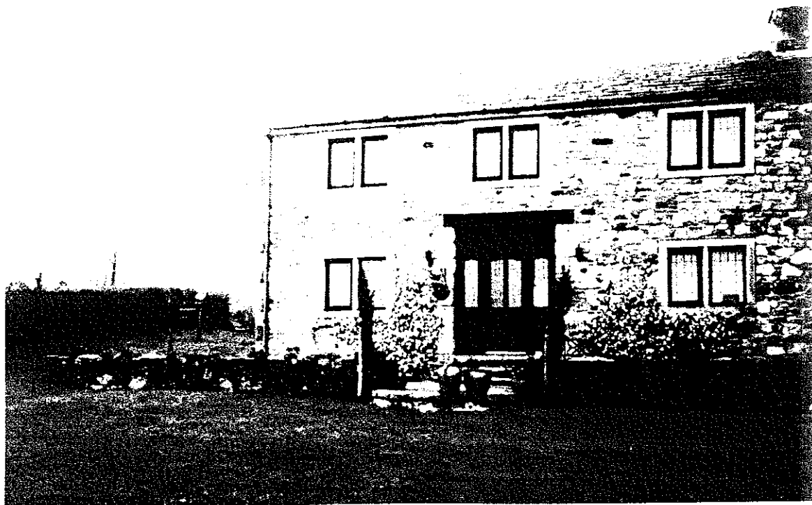
RYEPHILL GATE 8 new windows with white frames, 2 new windows regular new windows, for last 20 years, treatment
