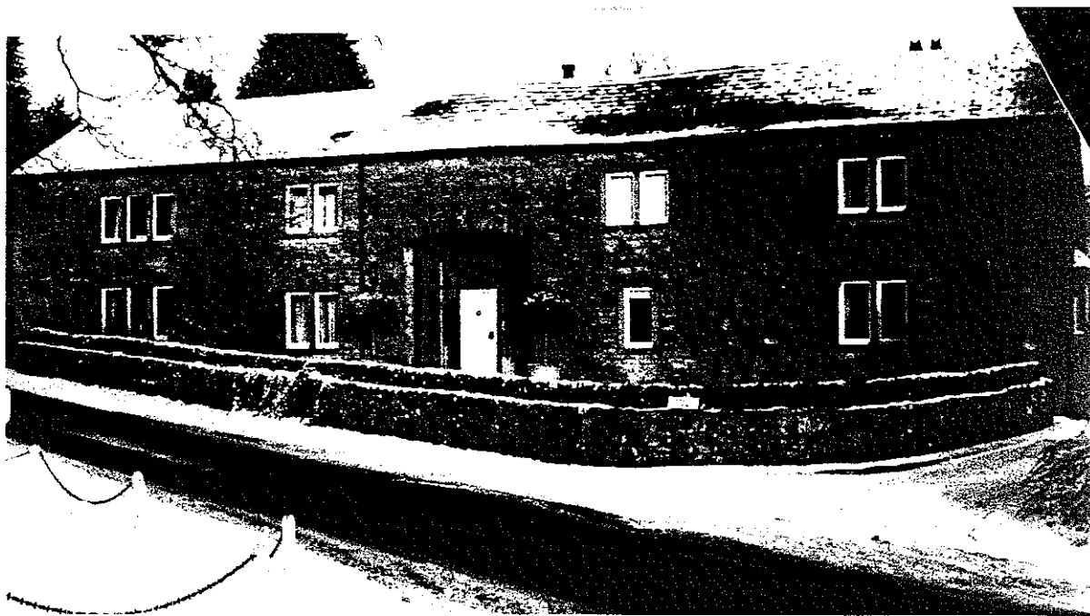
BRICK IN 1875 NEWTON village Centre several new regularly spaced new windows on both stories.
