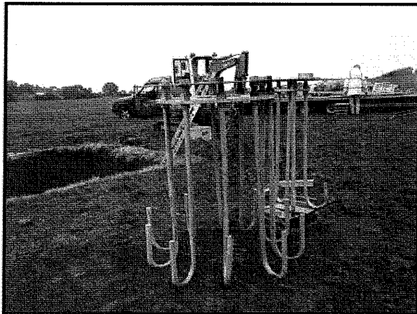
Typical reinforcement bars
