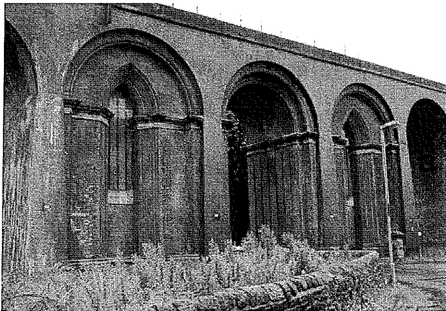
Whalley Viaduct 'gothic arches'
