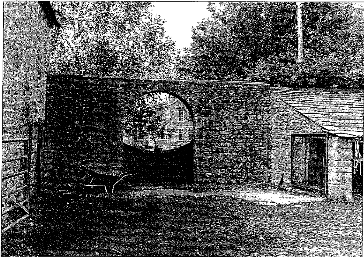
Photo 8: Garden wall to east of barn
