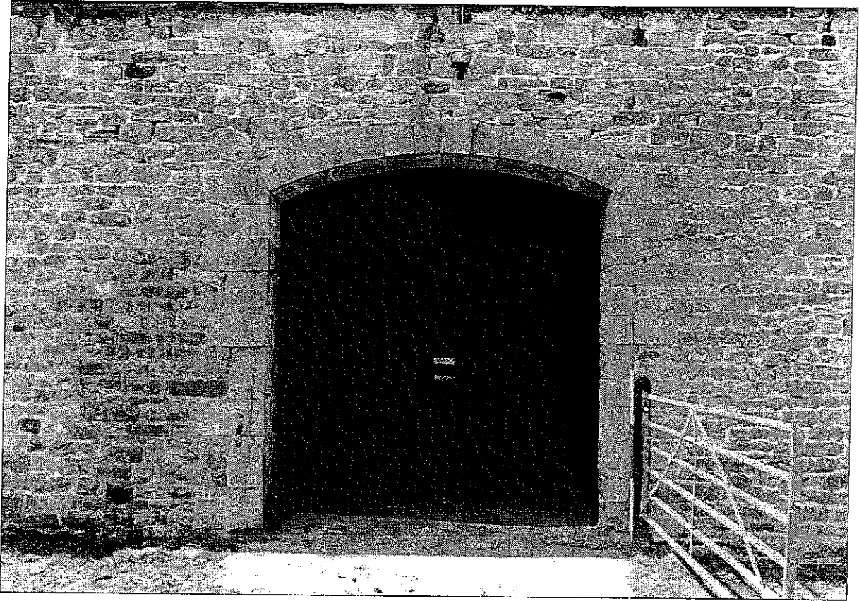
Photo 5: Barn: cart entrance
