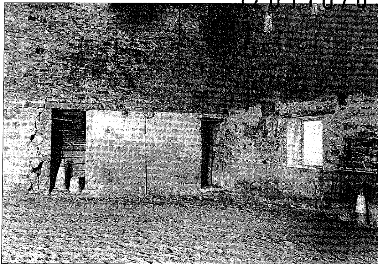
Photo 19: The barn: former shippon in north-west end
