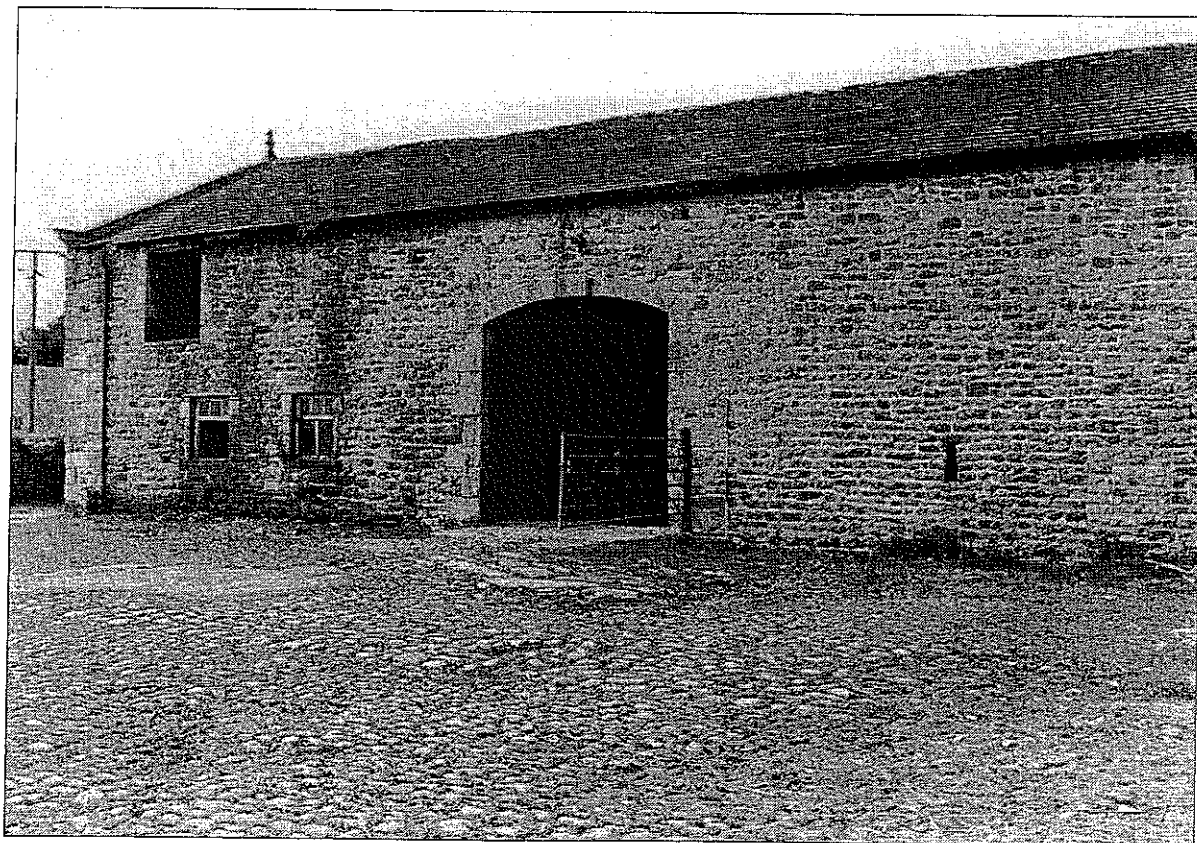
Photo 4: The barn, from the north
