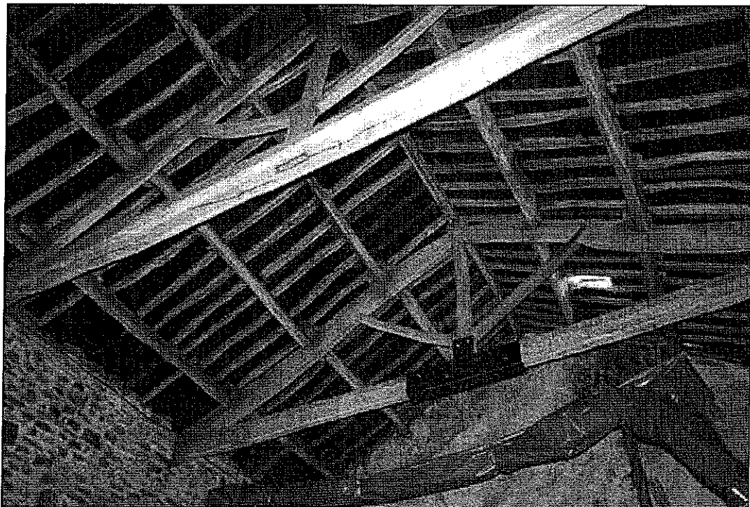
12. Kingpost roof trusses above the barn
