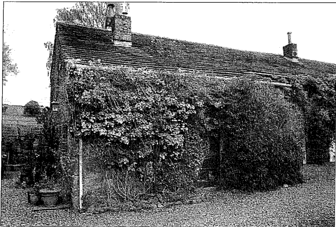
18. Southeast elevation, with modern glazed door
