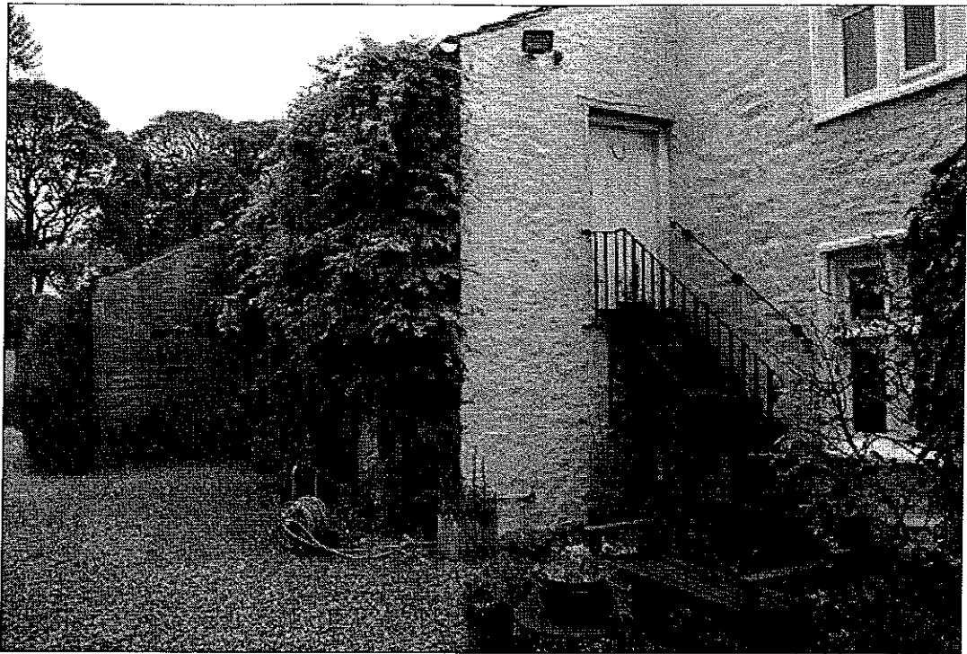
6 The barn, showing stable at junction with Rodhill Gate Farm. Rear of garage visible beyond
