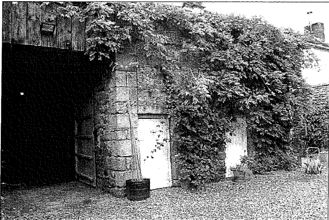
10 The stable joint by quoins of right wall of porch shows it is an addition
