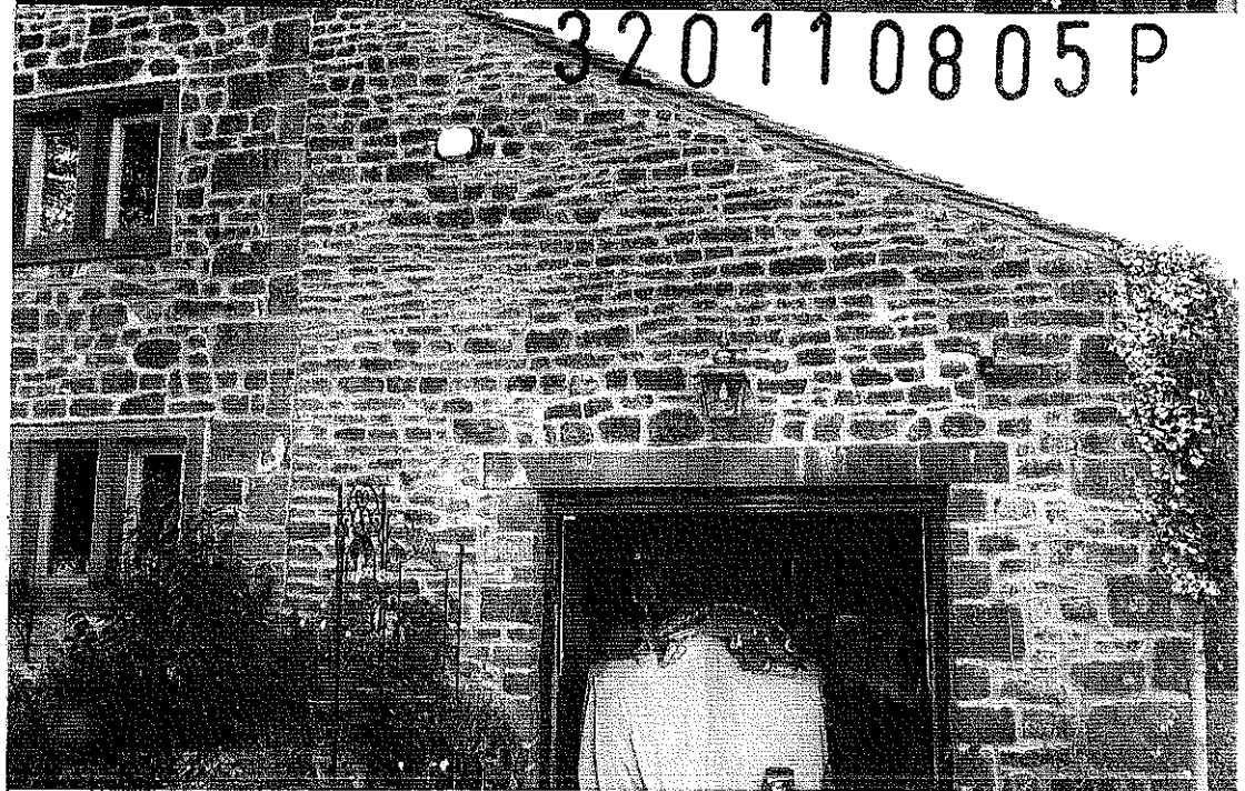
Photo 5 Existing Garage for proposed Conversion
