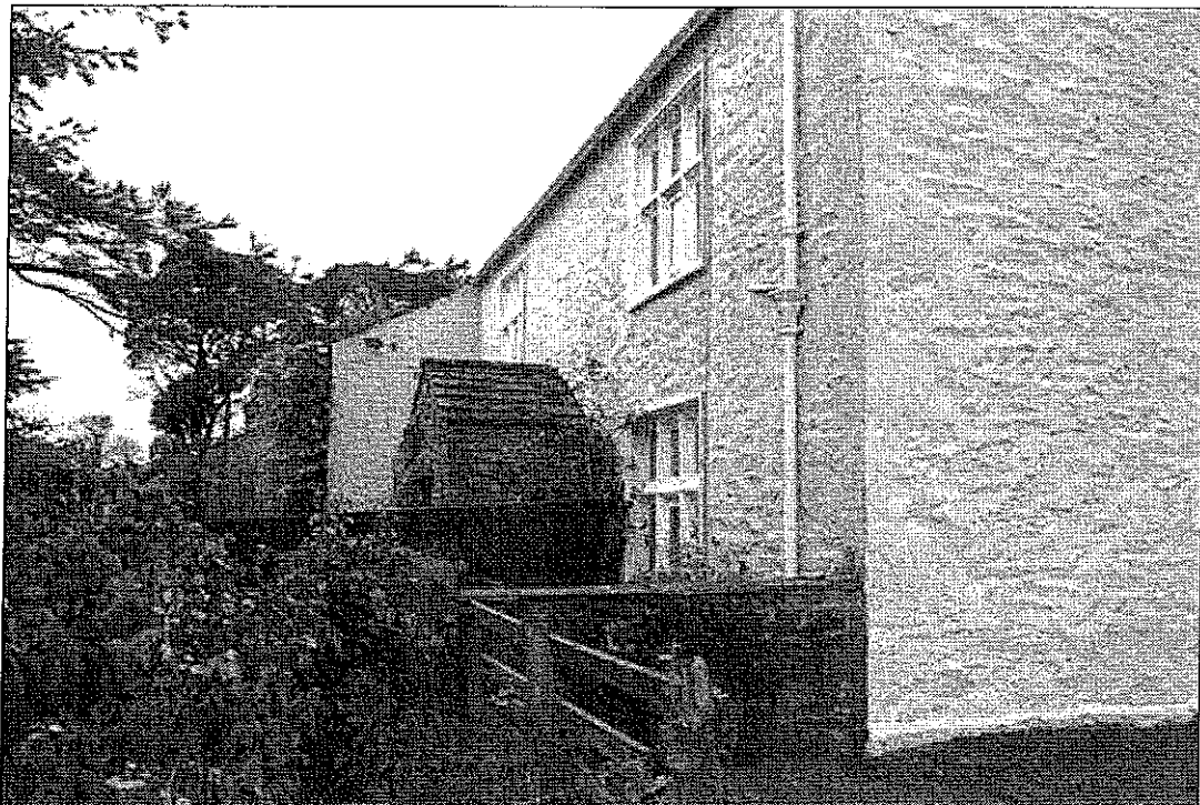
8. Rodhill Gate Farm looking southwest to the barn
