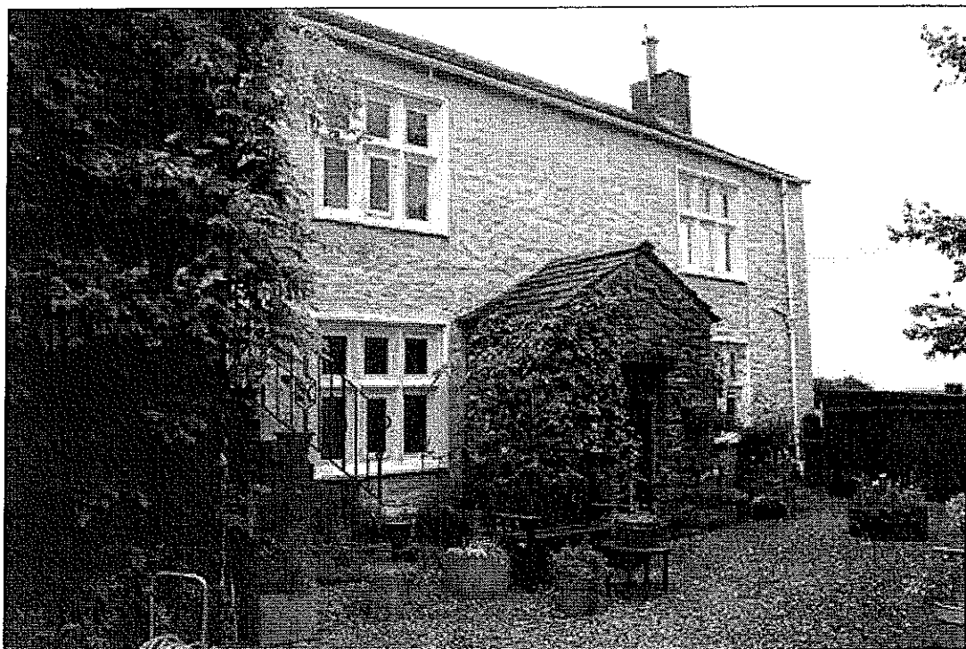
5. Rodhill Gate Farm from the south
