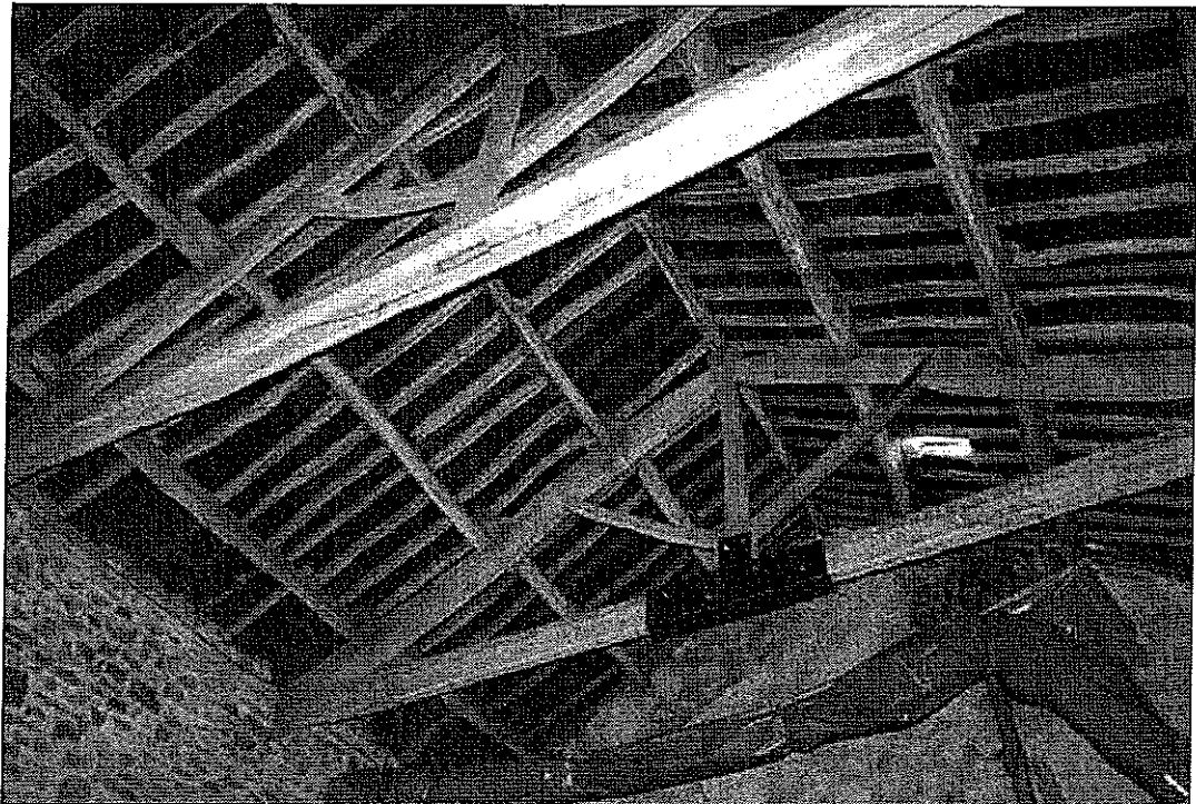
12. Kingpost roof trusses above the barn
