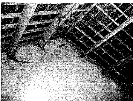
Figure 8: Barn B - roof detail
