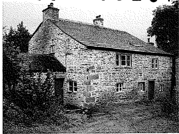
Blocked windows to right and left above door and below first floor windows.
